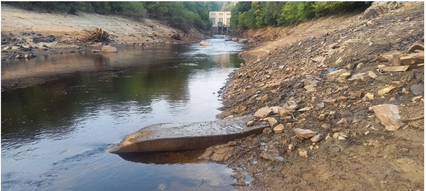
Blessington WWTP Discharge location in relation to Poulaphouca Power Station approx. 300 metres upstream. Between Poulaphouca Dam and Golden Falls Dam is now behaving like a pre Liffey Scheme river while work is being carried out at Golden Falls Dam.
