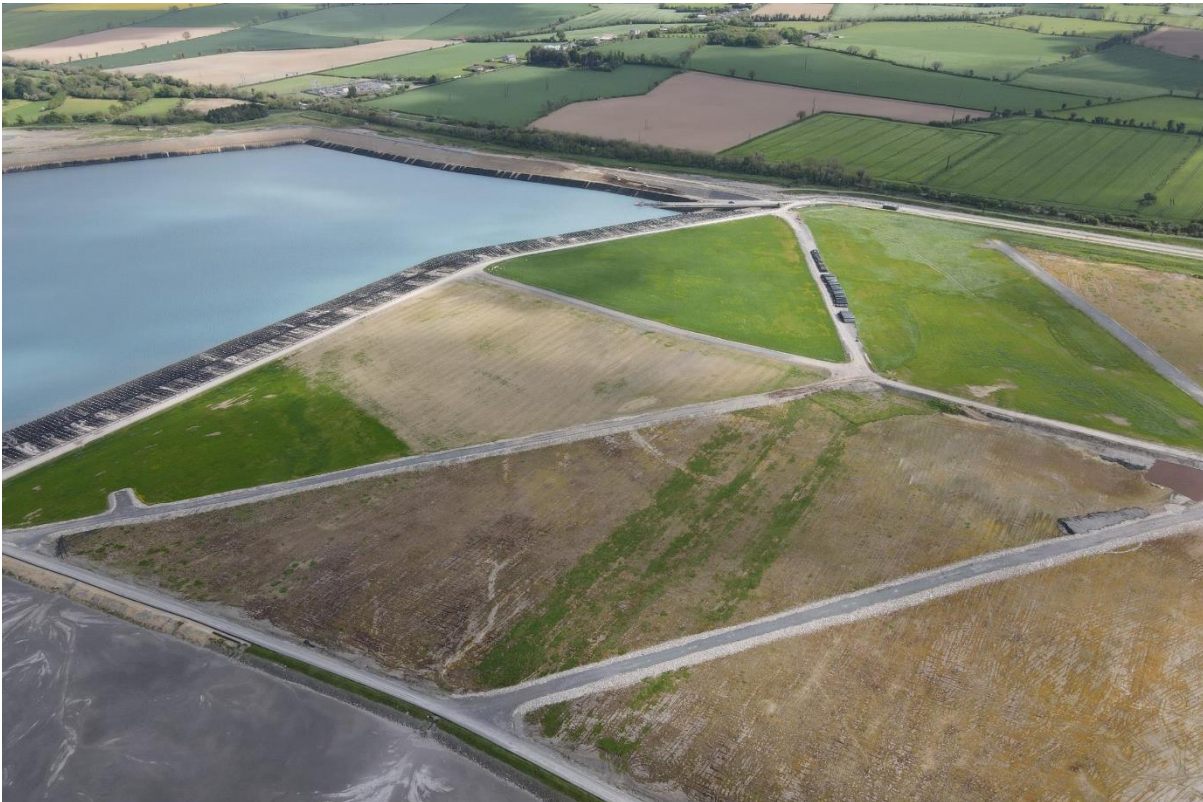
Figure 6-6 Capping trial Area in the Stage 5A north
