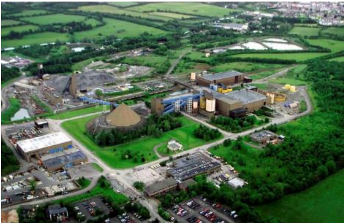
Figure 4-1 Overview of Knockumber Surface Site Facilities
