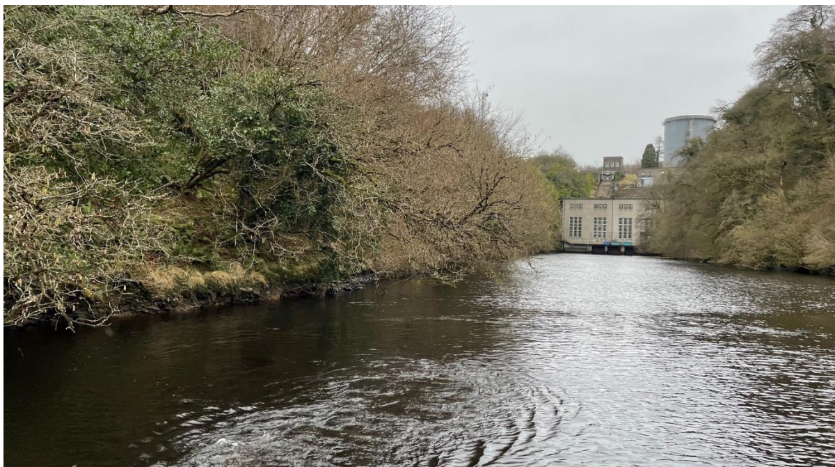
Over-hanging trees in narrow river section at Poulaphuca Station
