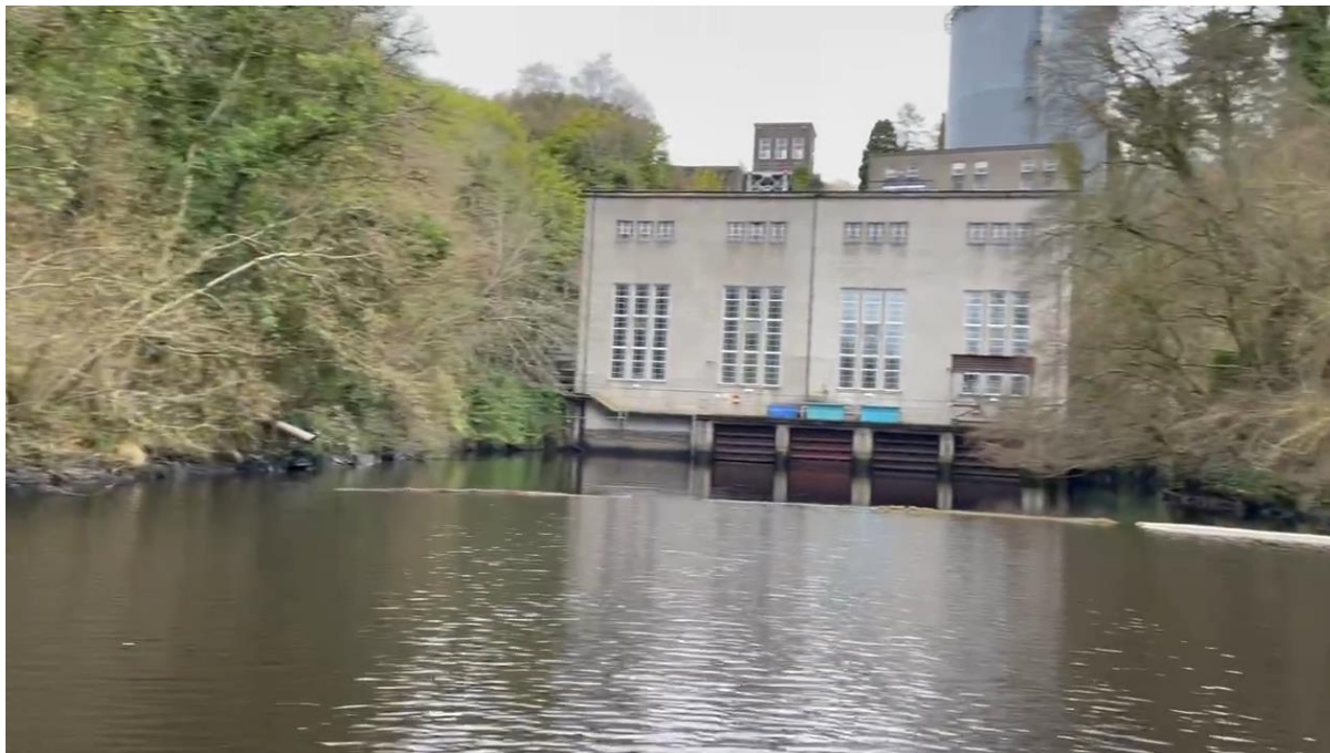
Boom across river at Poulaphuca Power Station
