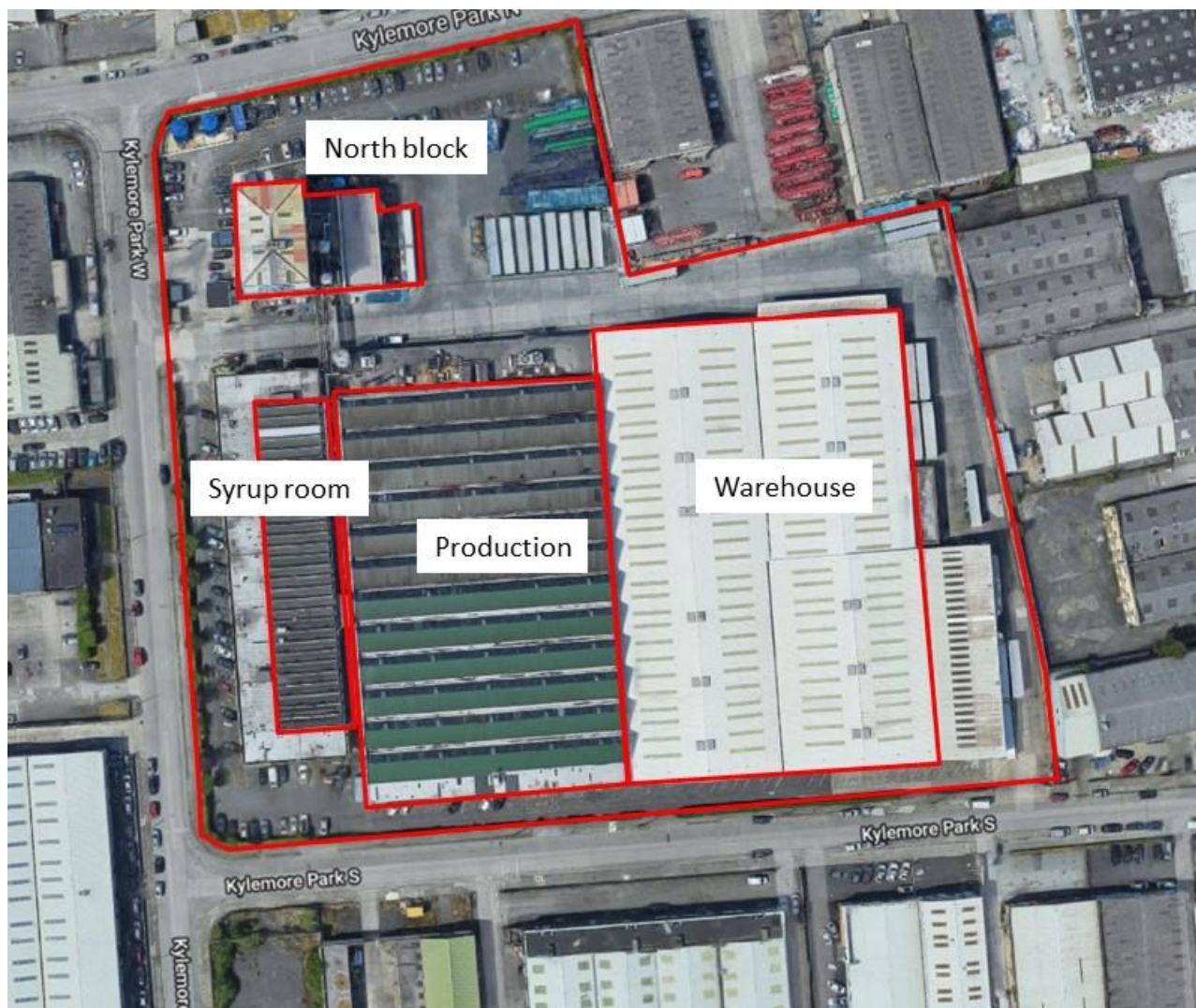
Figure 7-1 Kylemore Aerial View
