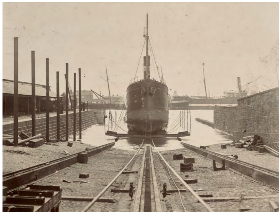
The SS Gale being hauled up Patent Slip No. 2, 13 April 1906 Source: Dublin Port Archive, ref 200212_10133
