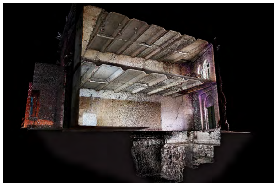
Laser scan survey showing the eighteenth-century sea wall under the redbrick substation at the junction of East Wall Road and Alexandra Road Source: ADCO for DPC
