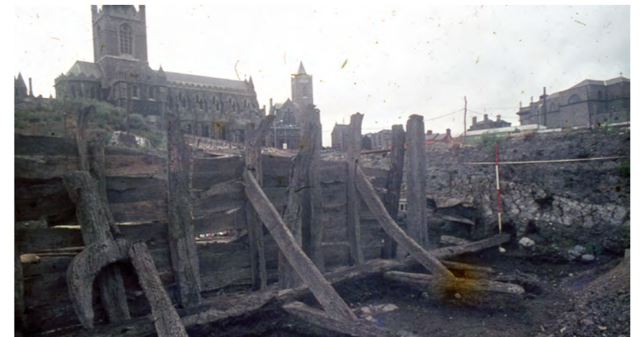
Wood Quay excavations showing river-front Source: National Museum of Ireland
