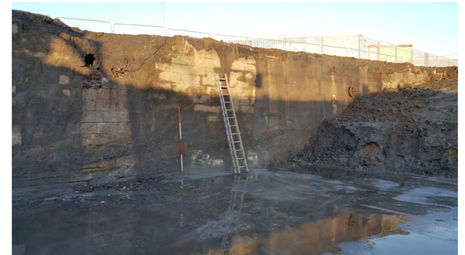
Patent Slip Quay under excavation, 2018 Source: ADCO for DPC
