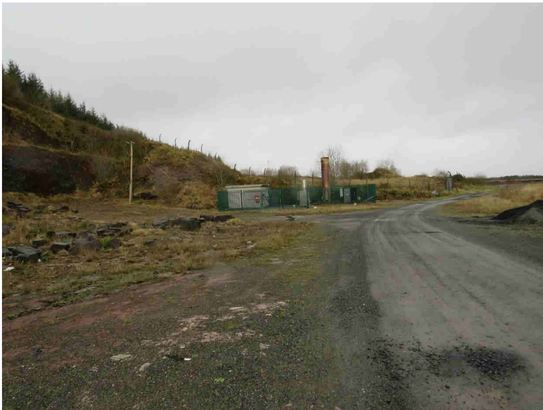
Figure 6.1. Buildings and artificial surfaces (BL3) located within the project site (28/01/22)
