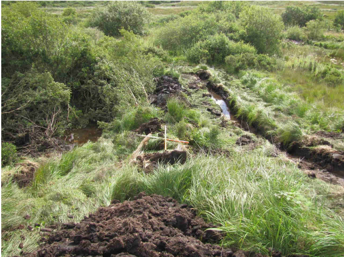
Plate 15. SE end of trenches 2 & 3 showing flooding in deeper peat.
