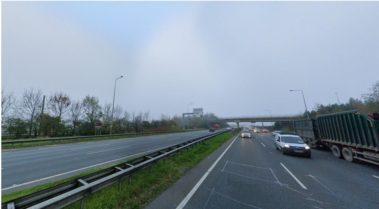
Plate 14-2: N7 National Road Westbound between J5-J6 Source: Google Street View Nov 2022
