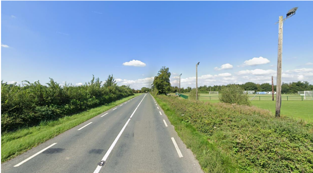
Plate 14-6: R403 Westbound Approach to Drehid WMF Source: Google Street View Aug 2021
