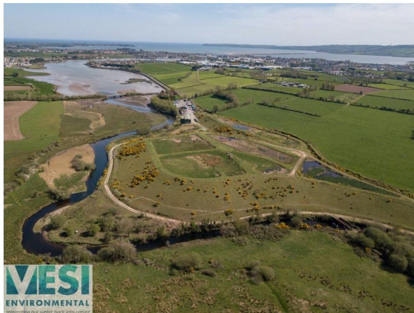
Figure 4. Dungarvan Landfill catering for landfill leachate since 2007, Co. Waterford.
