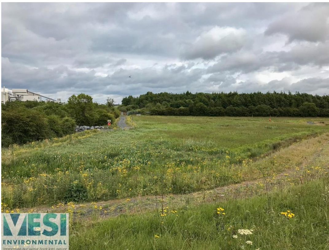
Figure 7: Roadstone Belgard Quarry ICW, catering for surface water runoff since 2016, Co. Dublin.
