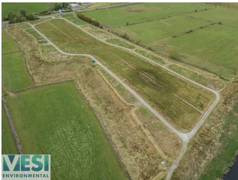
Figure 5. Churchtown Landfill ICW, catering for landfill leachate since 2014, Co. Donegal.
