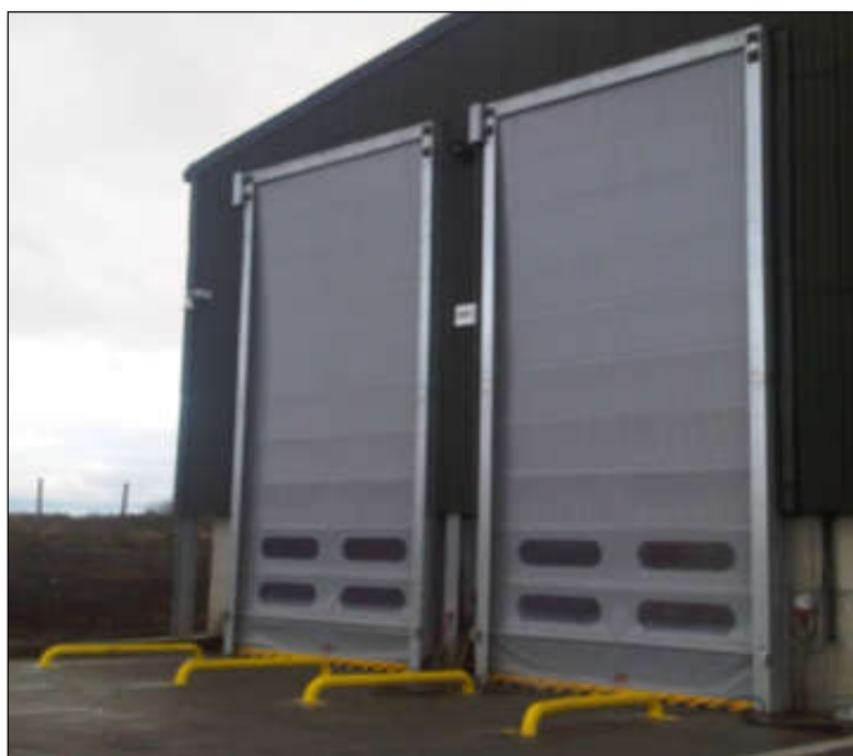
Figure 4-4: Image of waste receiving doors at existing compost plant
