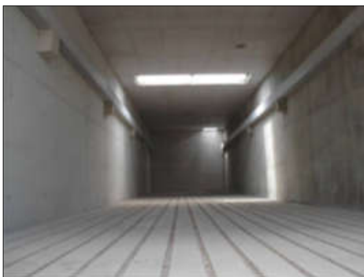
Figure 4-7: Typical composting tunnel with spigot floor
