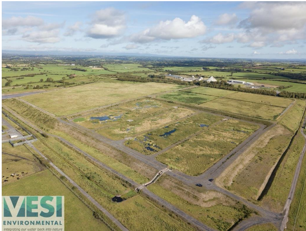
Figure 6. Galmoy Mines ICW, catering for Tailings Management Facility runoff since 2014, Co. Kilkenny.
