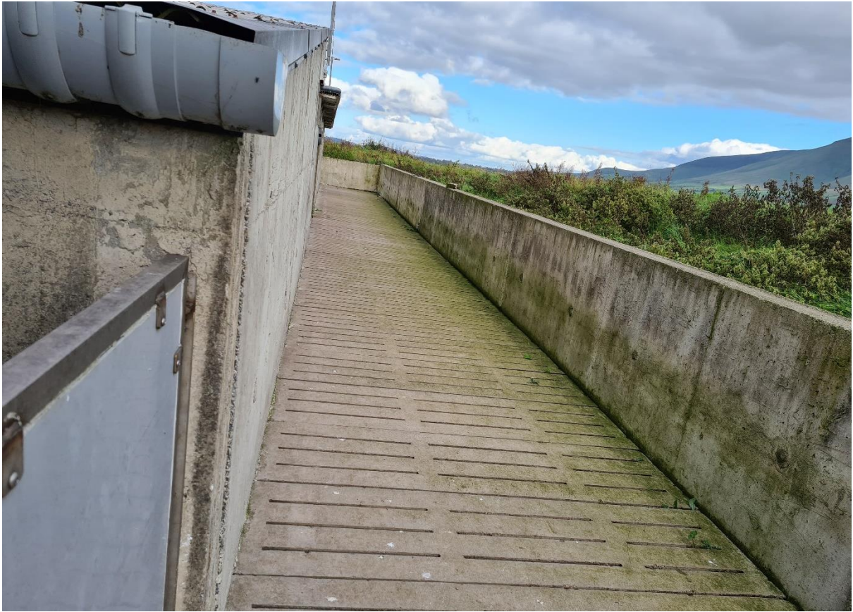
Plate 6: Un-covered slatted pig-walk passage.
