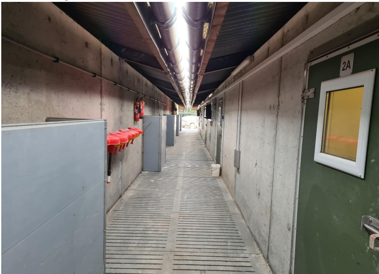
Plate 5: Covered slatted pig-walk passage.
