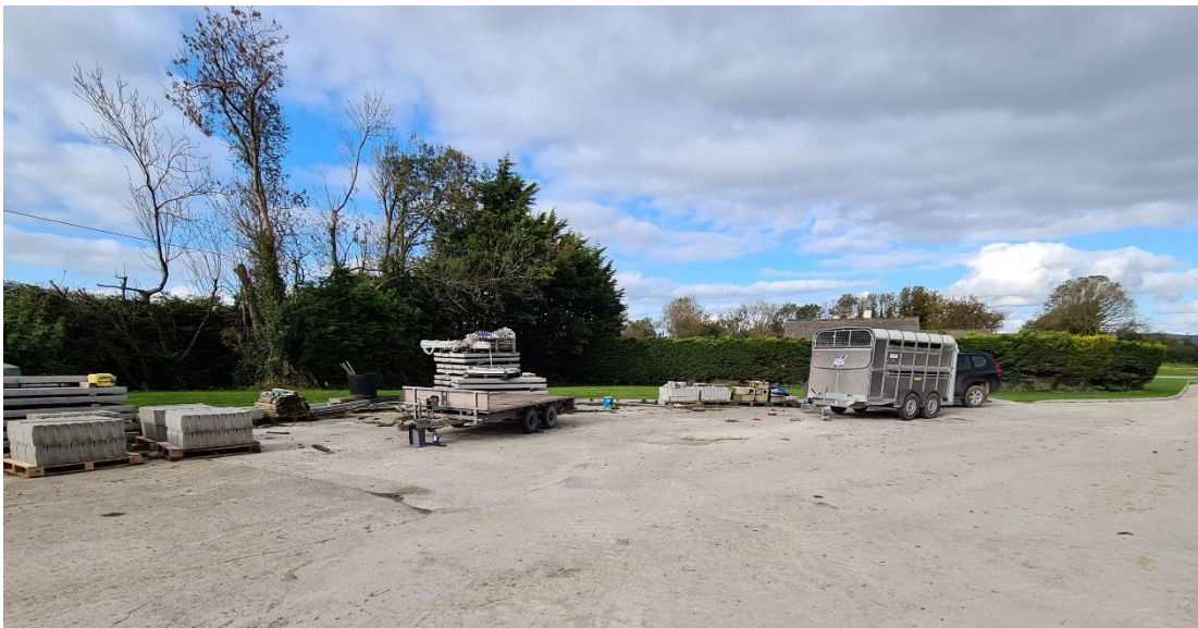
Plate 3: Site of proposed electrical substation
