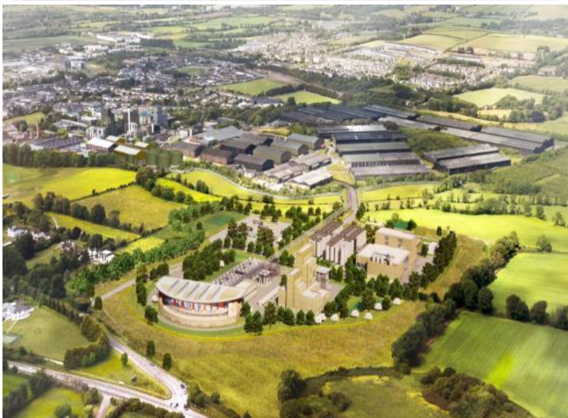
Overall site view
