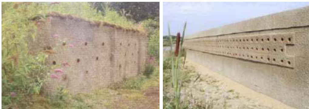
Figure 7-14 Example of artificial bank with Sand Martin nests (source: Hopkins 2001).
