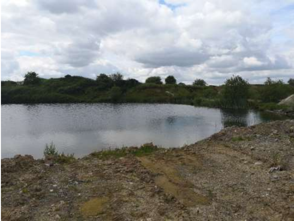
Figure 9-9 Settlement Pond in the southwest of the site
