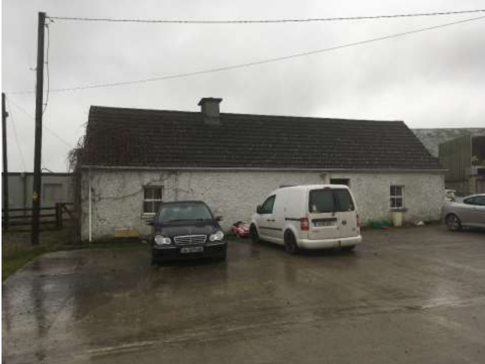
Plate 2: Vernacular cottage, facing southwest
