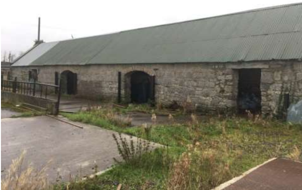
Plate 3: Vernacular outbuildings, facing northwest
