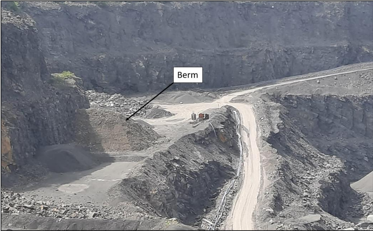
Fig. 1. Showing the beginning of berm construction.
