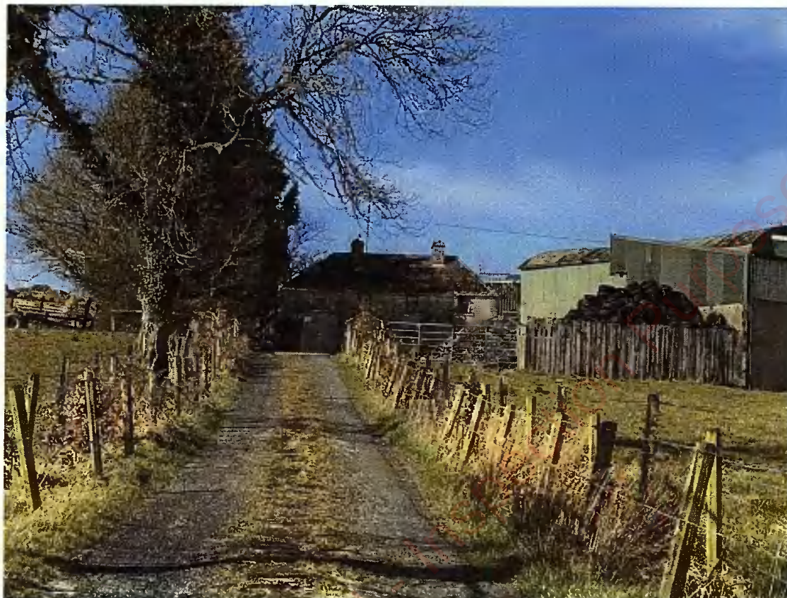
Existing structures on site
