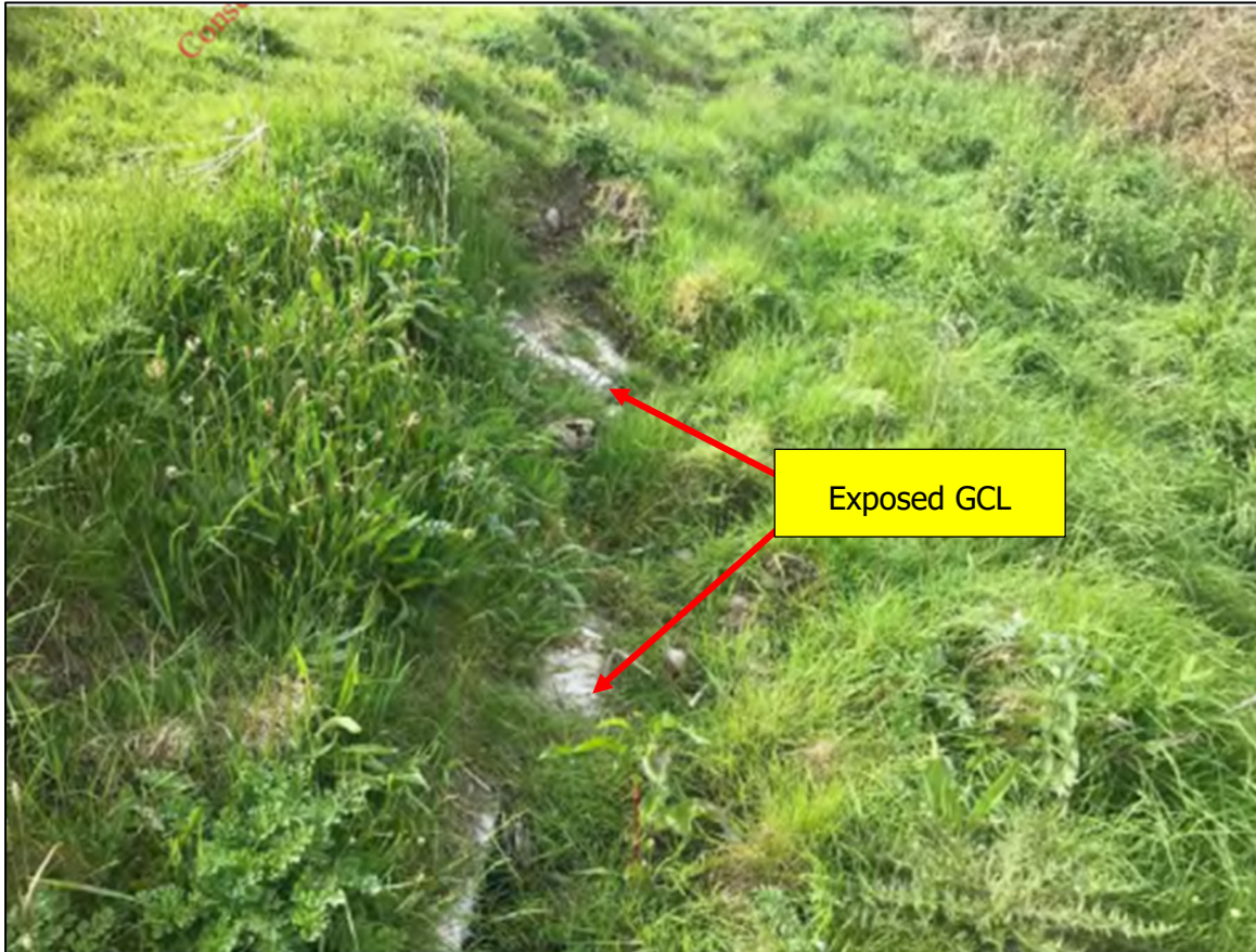
Figure 4: Exposed geocomposite clay liner (GCL)
