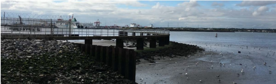
Figure 4 – Curved CWC outfall weir structure
