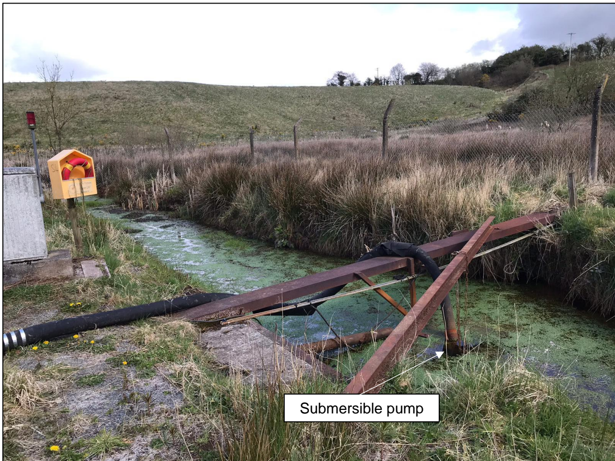
Figure 15 S4 pond (foreground) and landfill (background)
