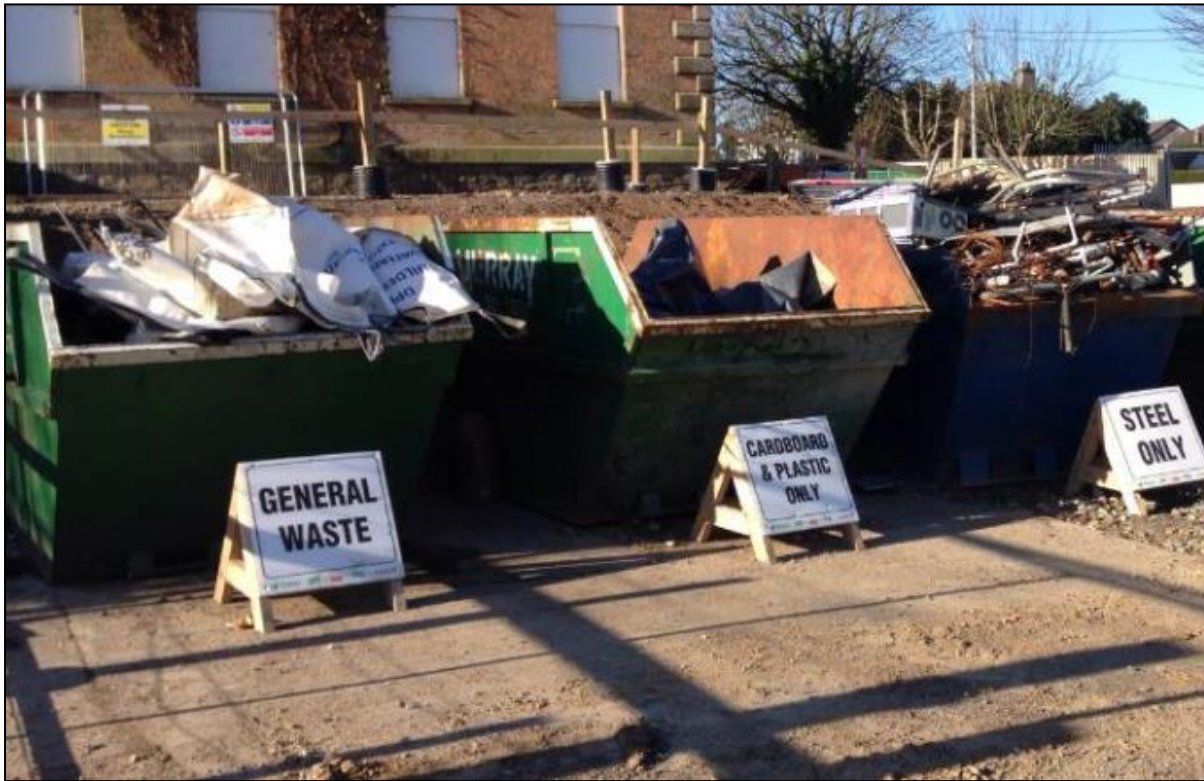
Example waste segregation arrangement using skips.
