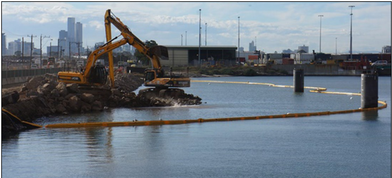
Figure 16 Example silt curtain arrangement surrounding dredging activities.
