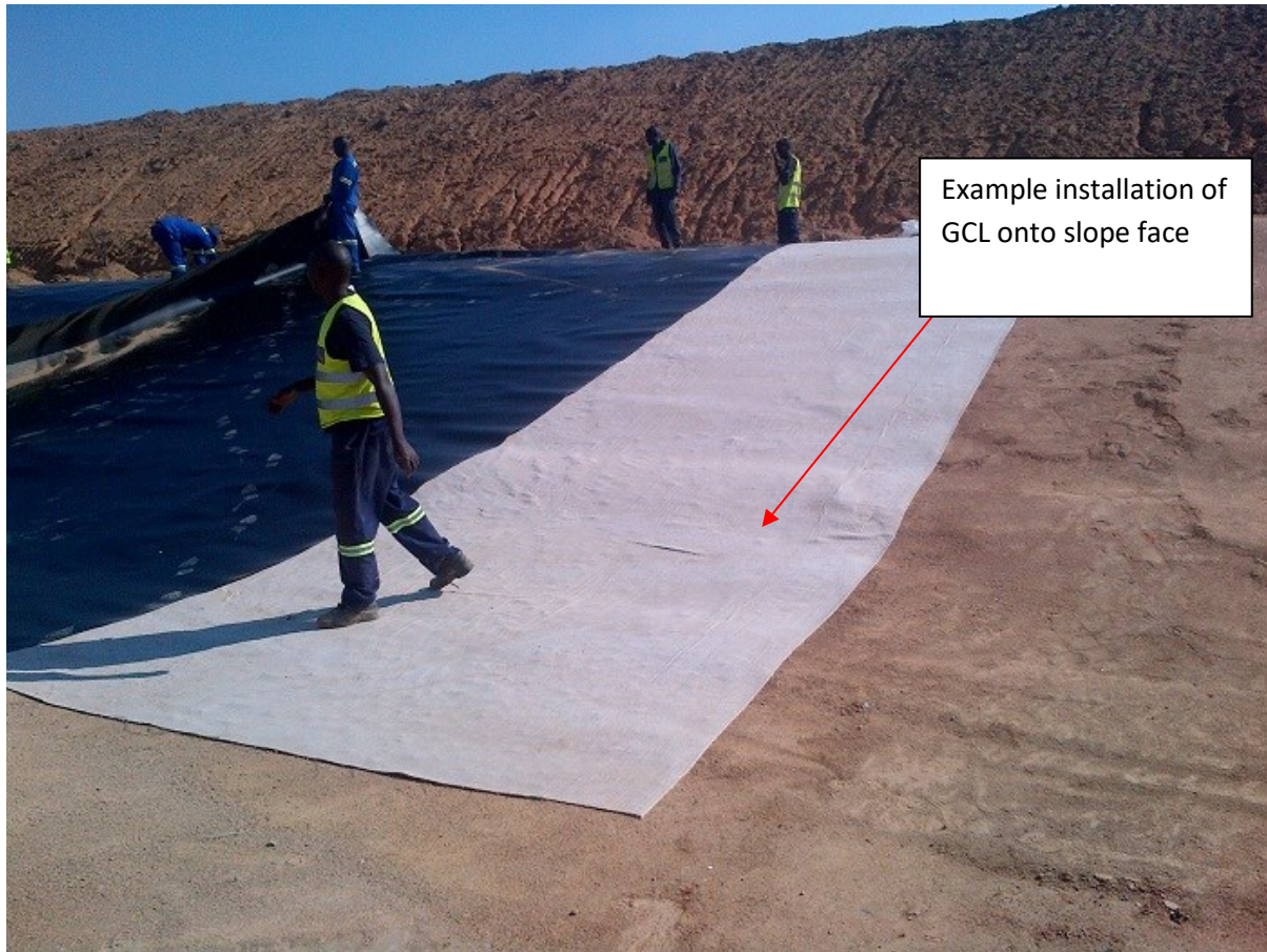
Figure 13 Showing a typical clay liner installation process.
