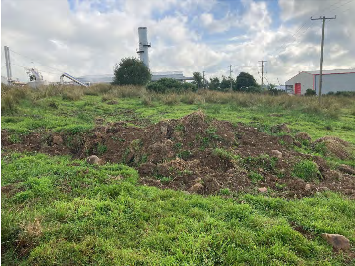
Figure 11-6 Development site showing engineering test pit
