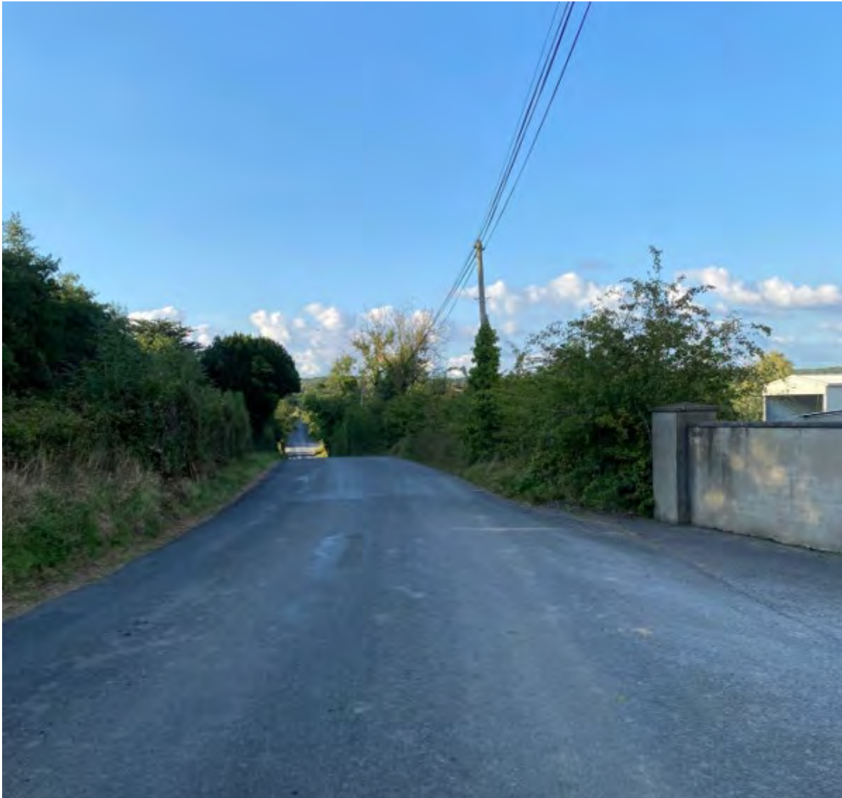
Figure 12-3: College Road looking north – typical vertical and horizontal alignment (source: SRC)
