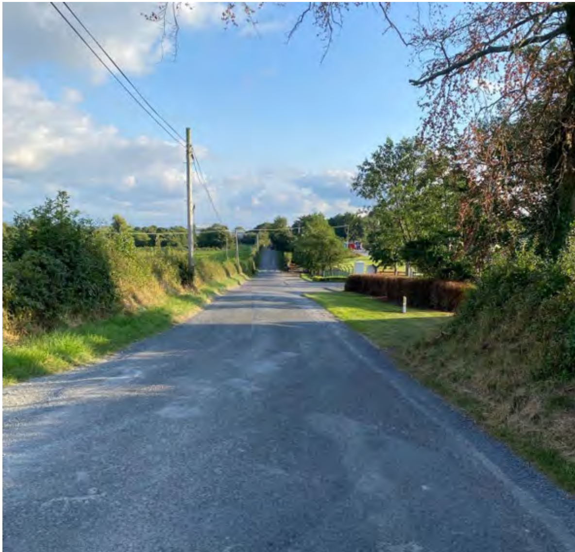
Figure 12-6: Southbound forward visibility of College Proteins access (source: SRC)
