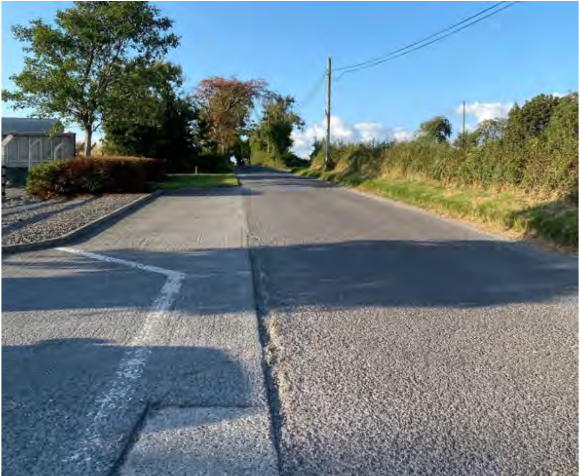
Figure 12-4: Existing sightline +150m to left from College Proteins access (source: SRC)
