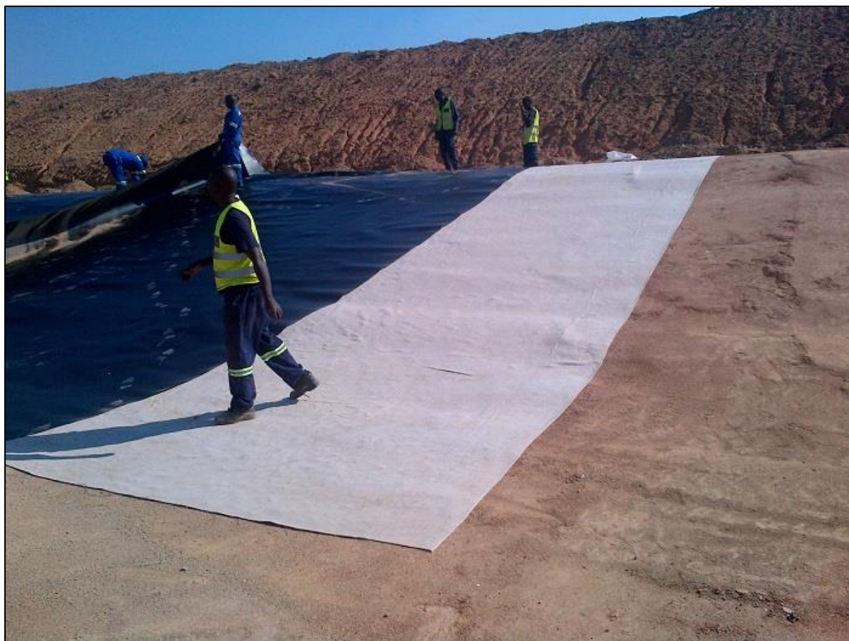
Figure 13 Showing a typical Geosynthetic Clay Liner (GCL) installation process.
