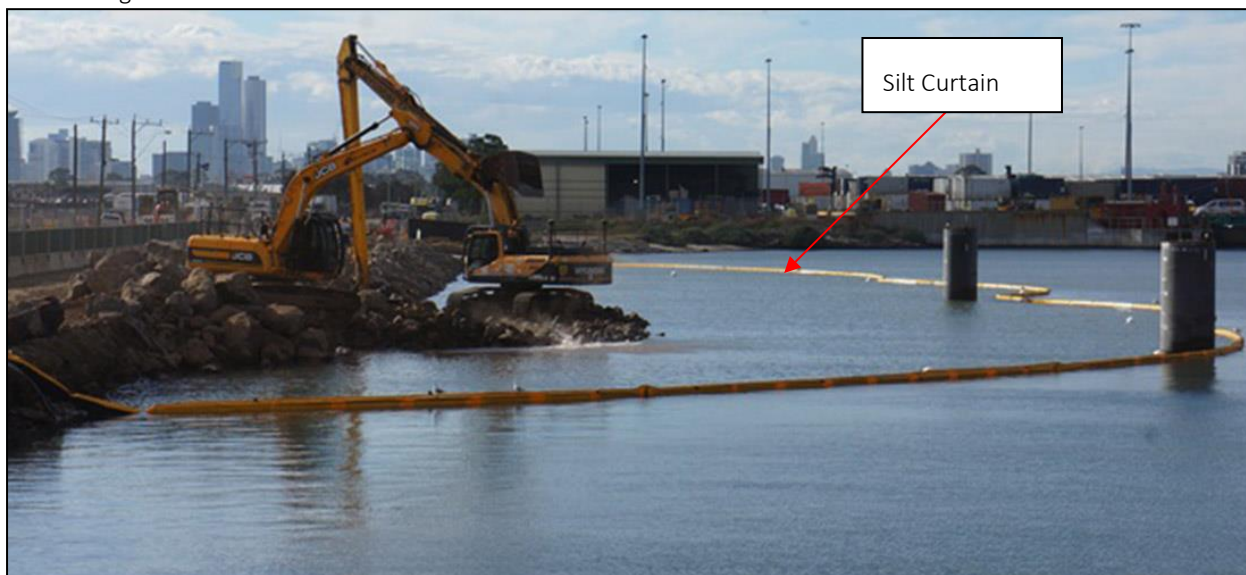
Figure 18 Example silt curtain arrangement surrounding dredging activities.
