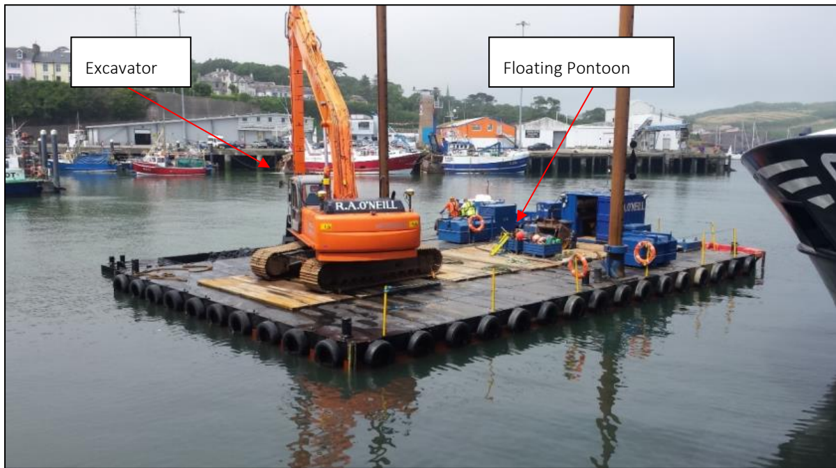
Figure 1 Example dredging operations using a floating barge and long reach excavator.
