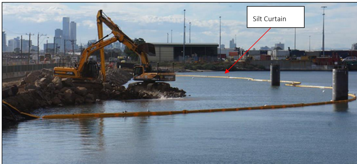
Figure 3 Example silt curtain arrangement surrounding dredging activities.
