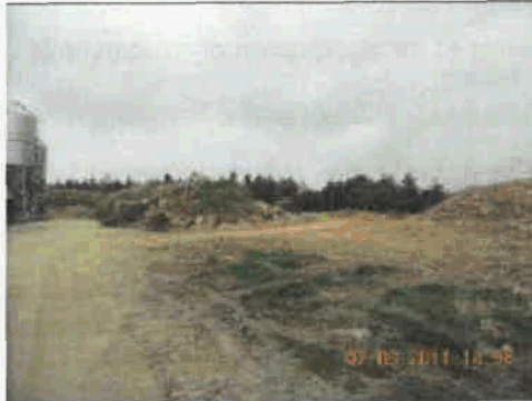
access road created at north-eastern section of site
