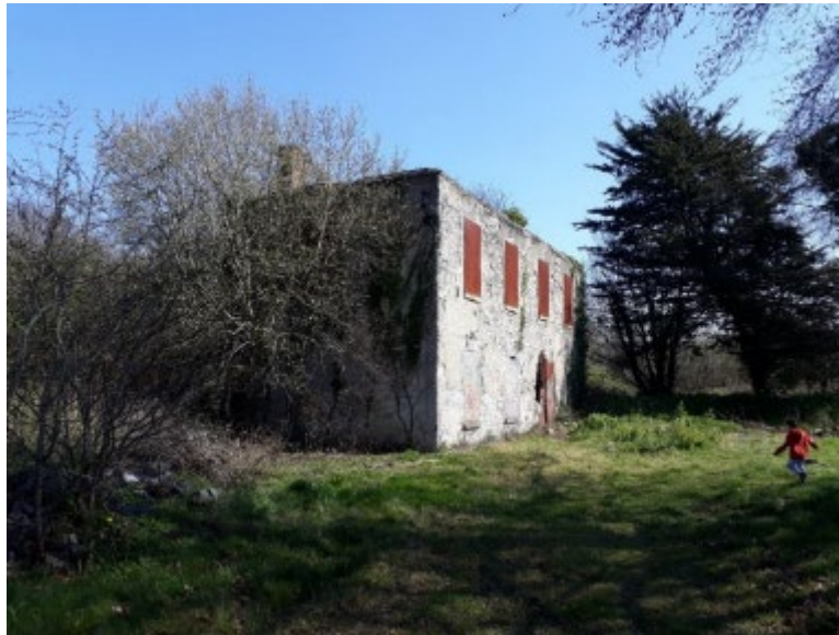
Derelict farmhouse close to river Liffey with potential for future development
