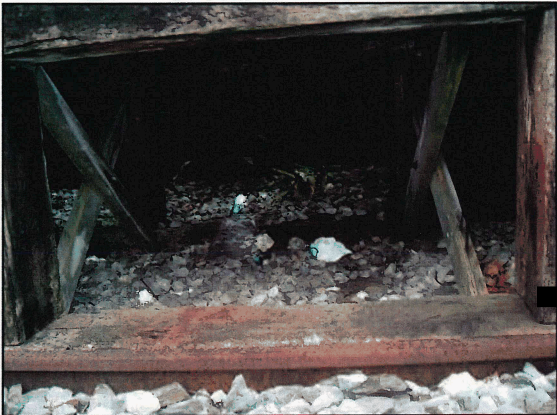
Photos showing Hard Core Gravel Fill in front of Model Railway Building
