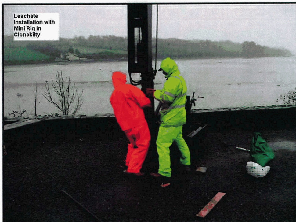
Installation of Leachate Well No.5
