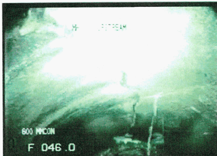
Photo: 12a, Tape No.: 1, 0000 46.7m, Multiple Cracks, from 11 to 01 o'clock
