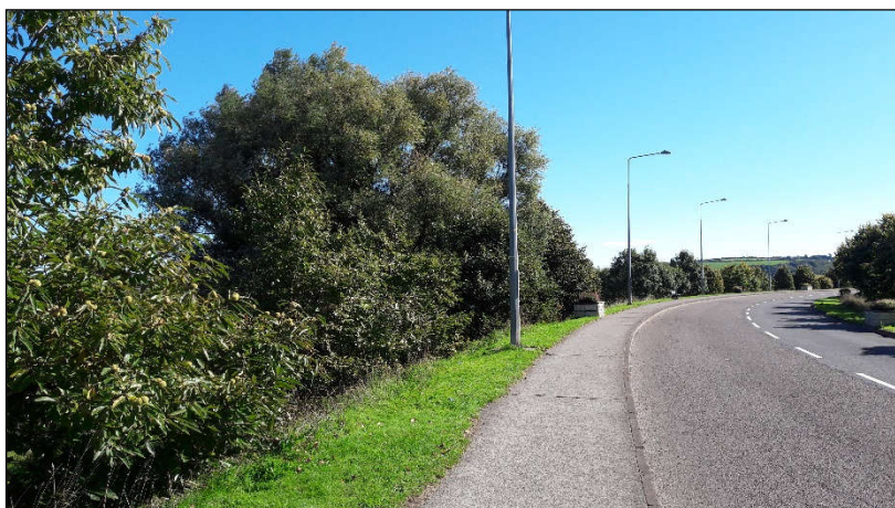
Plate 10-14 - Treeline relief road (2) – looking east.
