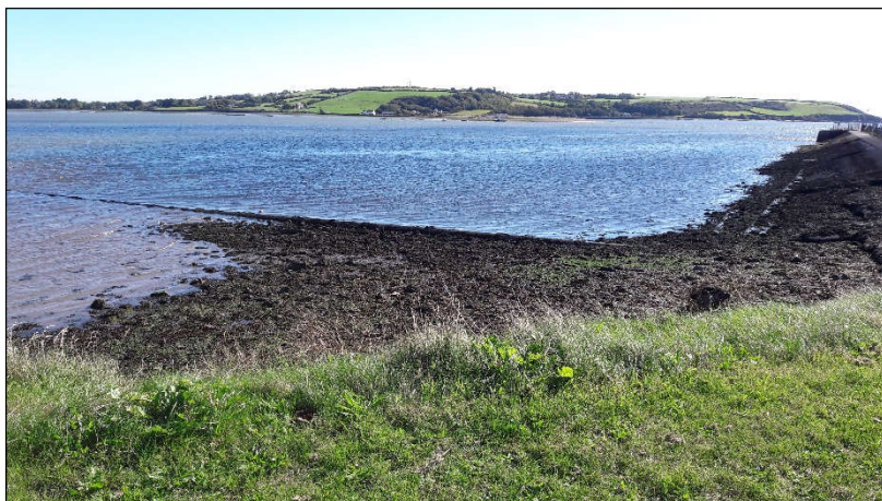
Plate 10-19 - Dunn's Park outfall pipe.
