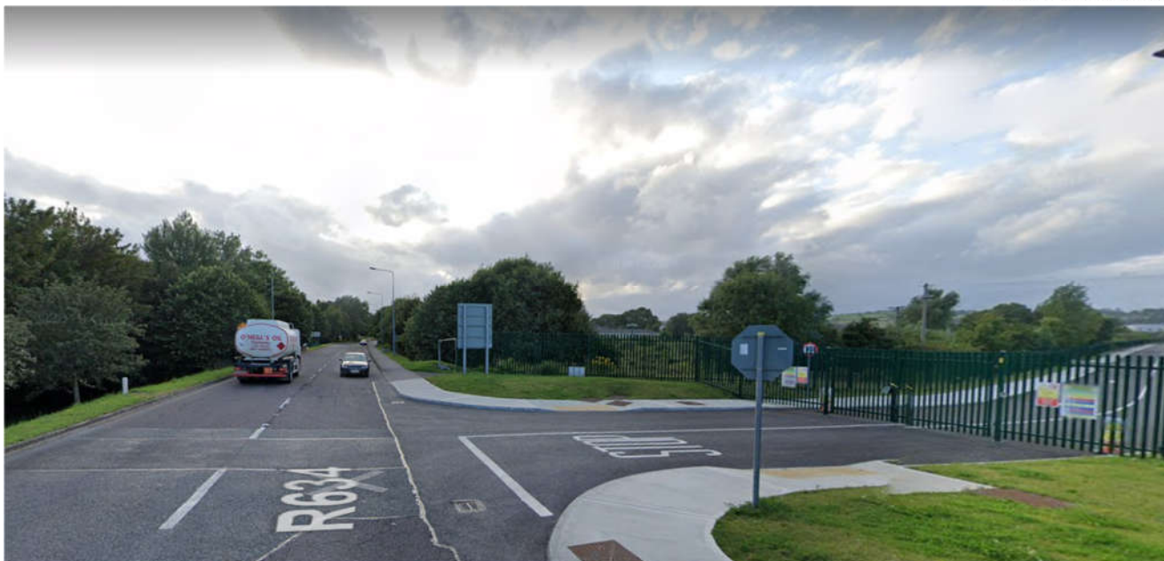
Plate 7.1: Existing WwTP Access
