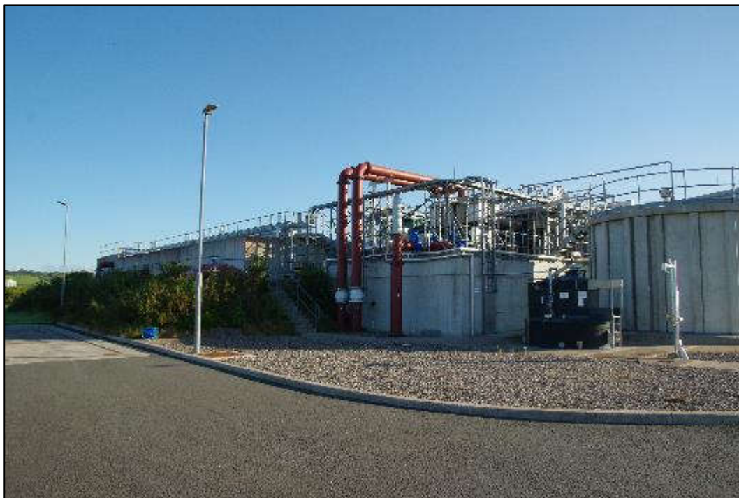
Plate 8.1 - View of existing infrastructure within WwTP
