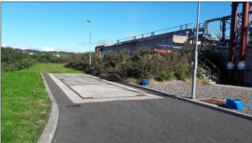
Plate 10-2 - Berm around the WWTP, heavily overgrown with gorse.
