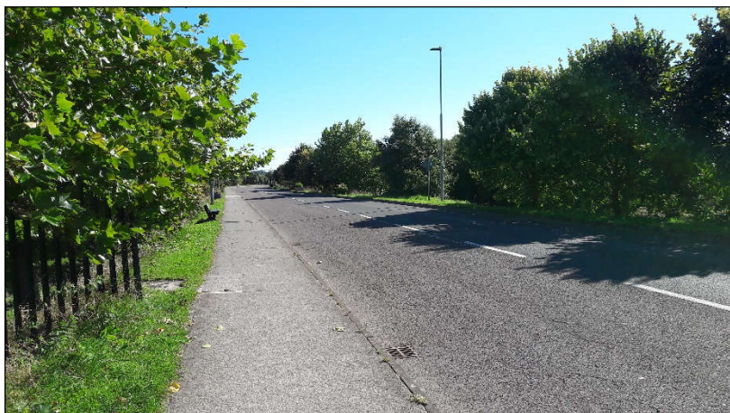
Plate 10-13 - Treeline relief road (1) – looking east.
