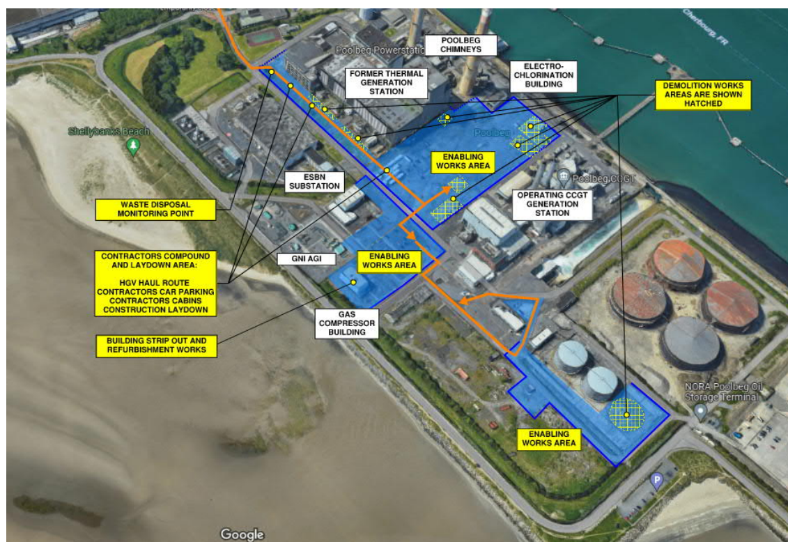
Figure 3.5: Aerial View of ESB Poolbeg Generating Station looking Northwest showing the Extent of the Proposed Demolition & Enabling Works
