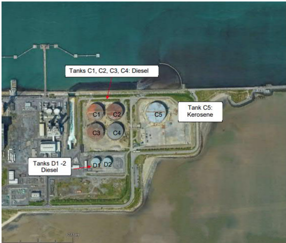
Figure 5.6: NORA Fuel Tanks
