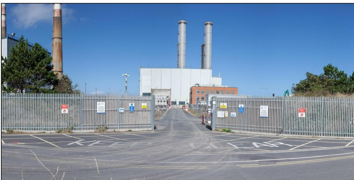
Figure 13.4: Vehicular Entrance to the South of the Site
