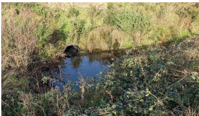
Figure 5.21 Anngrove Stream at Road Culvert
