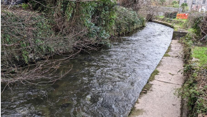
Photo 5 Dungourney River at SW016/SW018/SW021
