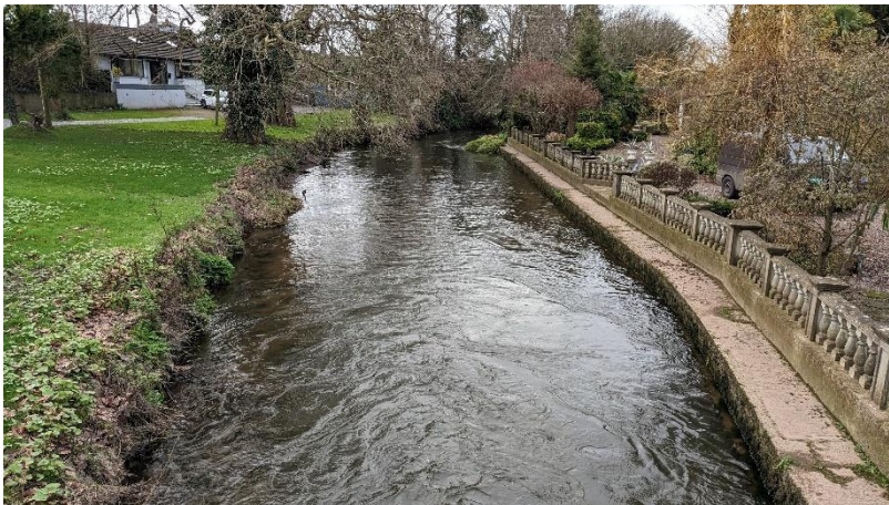
Photo 6 Midleton Bridge u/s SW017
