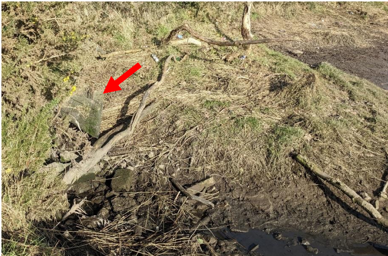
Photo 8 Outfall at SW020
