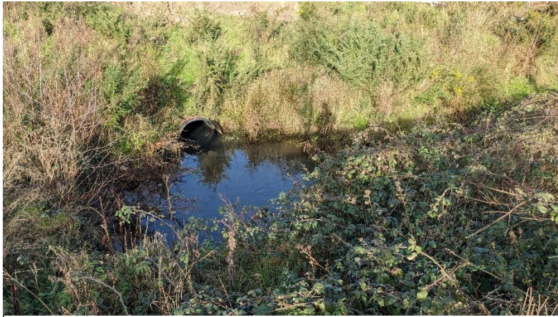
Photo 18 Anngrove Stream at road culvert
