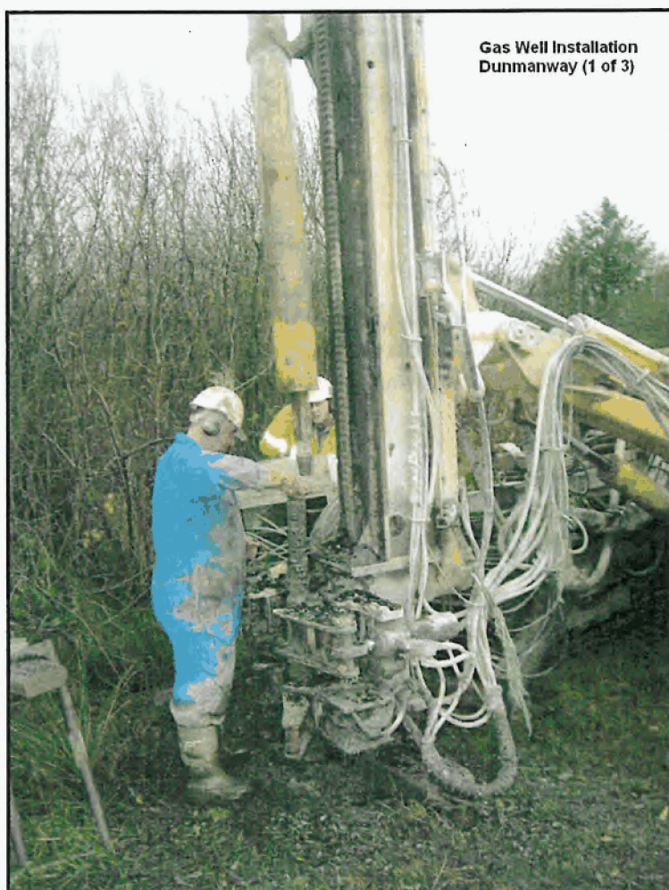
Installation of Gas Well No.2
