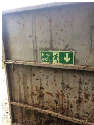
Plate 4: Fire Exit in Shed 3
