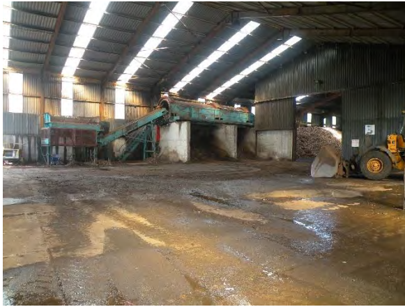
Plate 3: Screened Material Storage
