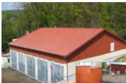
BEKON Kusel on Farm Biogas Facility
