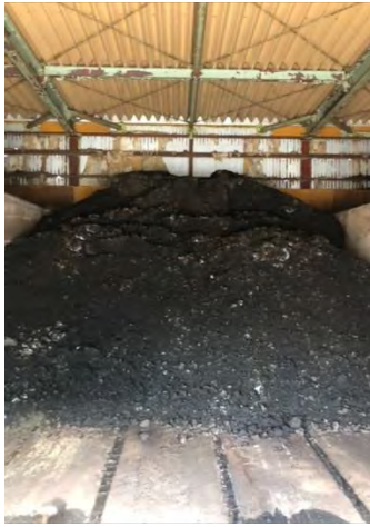
Under-floor Forced Air System
