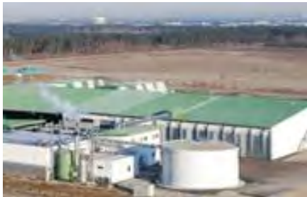
BEKON Munich Pilot Plant
