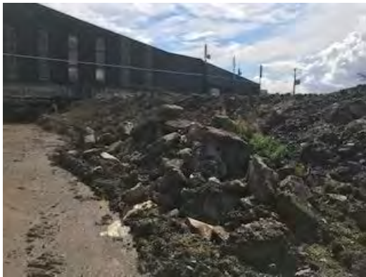
Plate 8-3: Soils Beneath Old Shed to South
