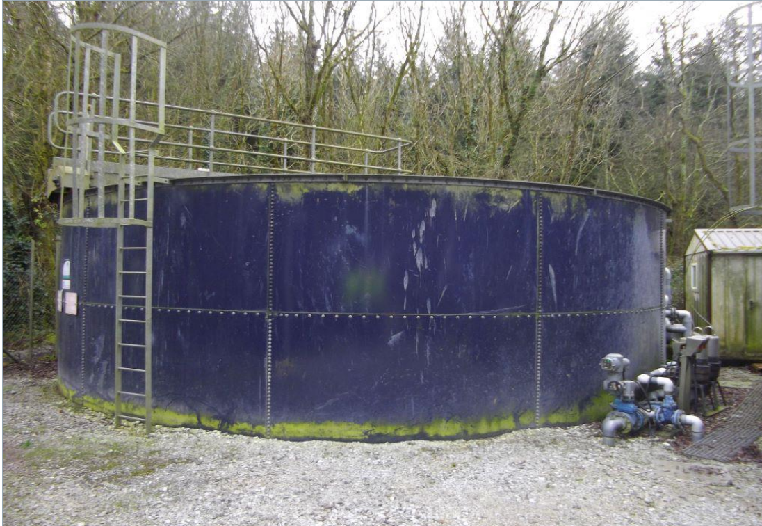
Figure 2.4: View towards existing clarifier tank located on the site.
