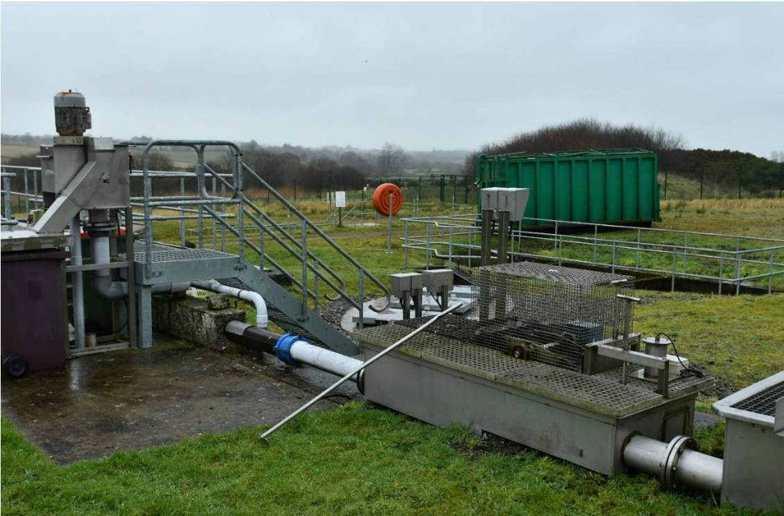
A2.1 Existing WwTP.
