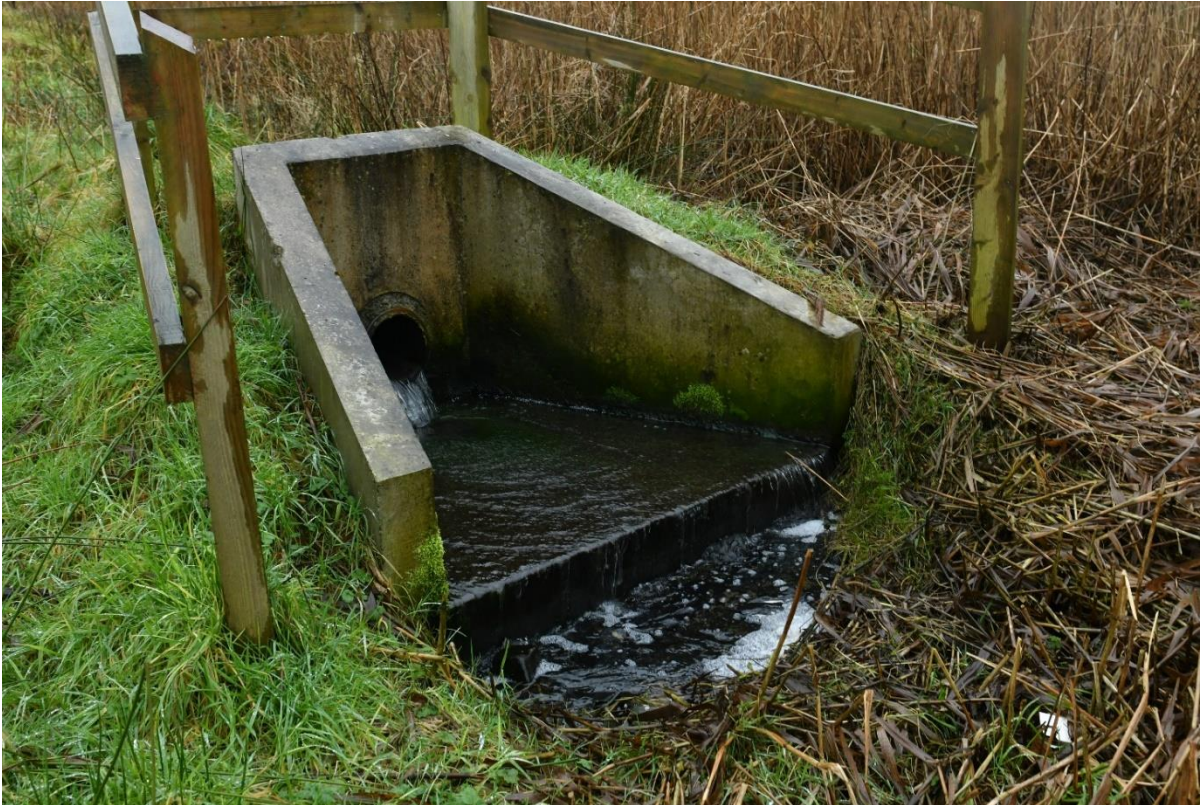
A2.7 Existing wastewater discharge point to channel leading to Brogeen River.
