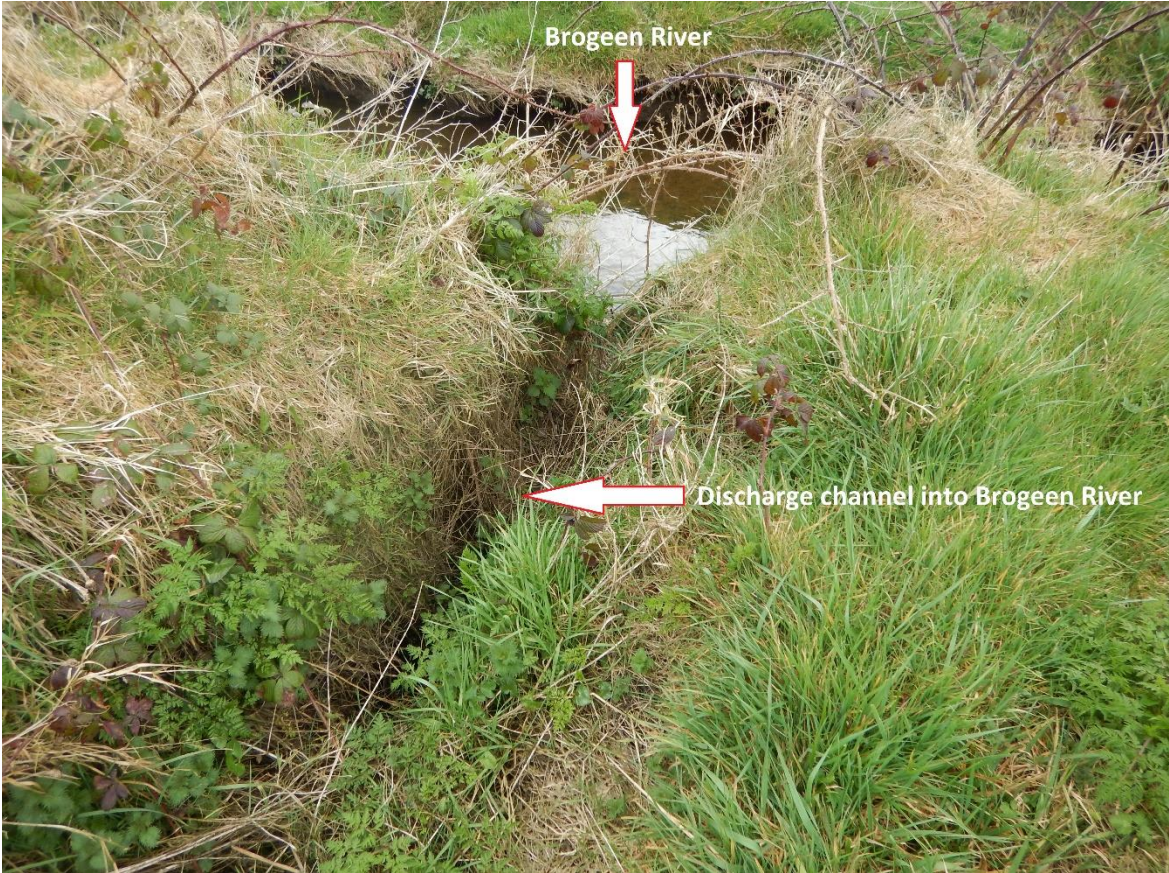
A2.8 Channel from discharge point into Brogeen River.
