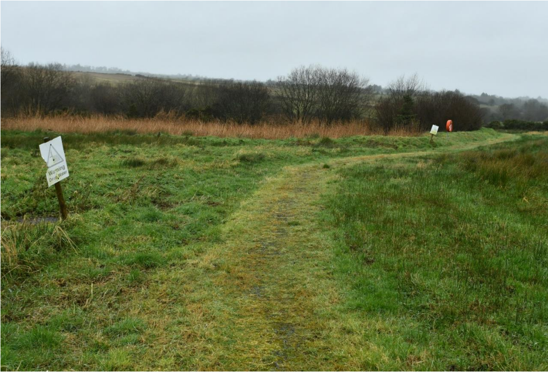
A2.5 Internal site access to constructed wetlands.
