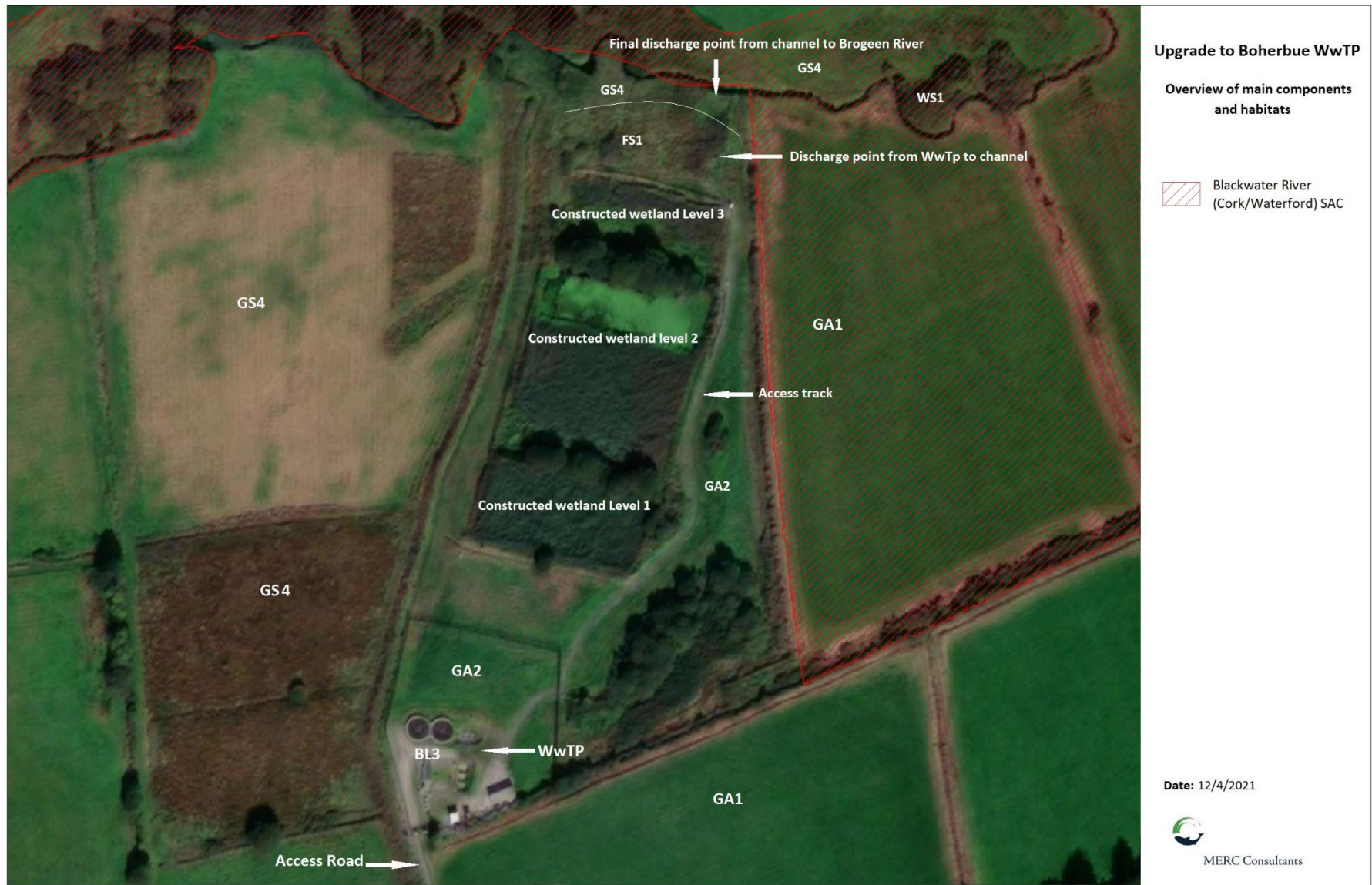
Figure 5.2. Existing site infrastructure and habitats
