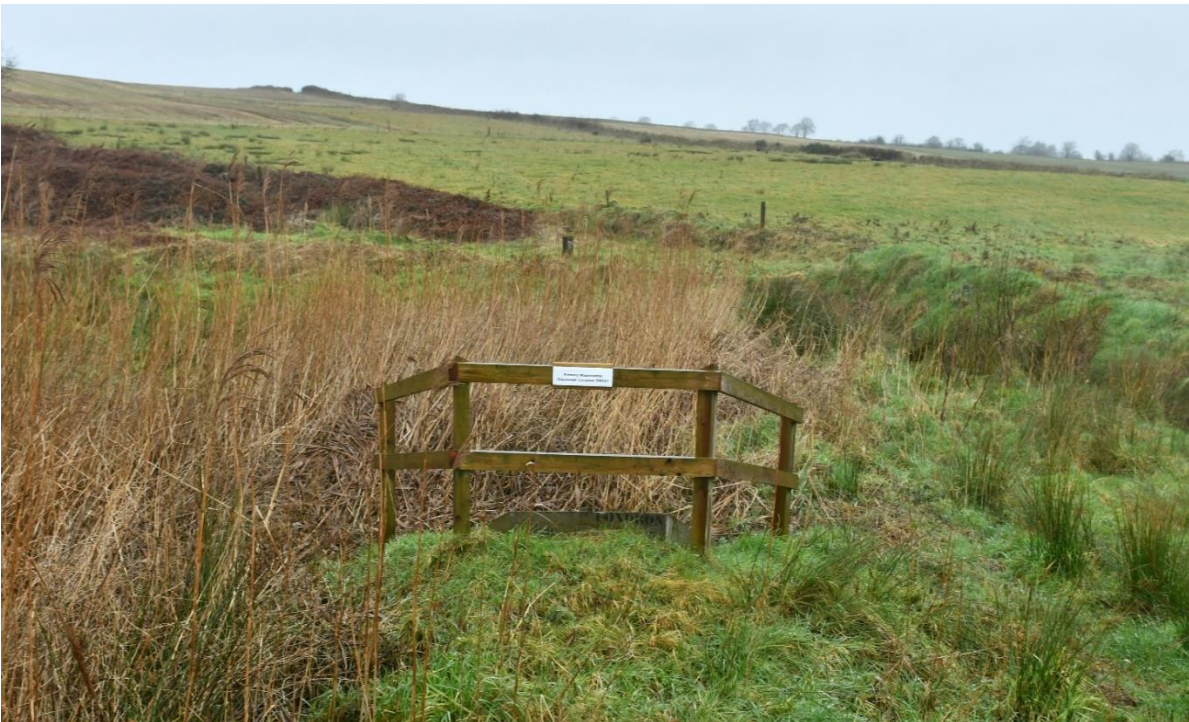
A2.6 Existing wastewater discharge point to channel leading to Brogeen River.
