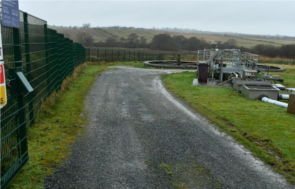
A2.2 Existing WwTP.
