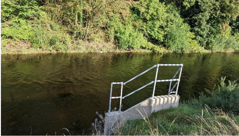
Photo 5 WwTP Primary Discharge SW001
