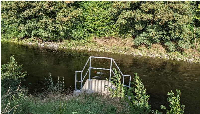
Photo 3 WwTP SWO/EO SW002
