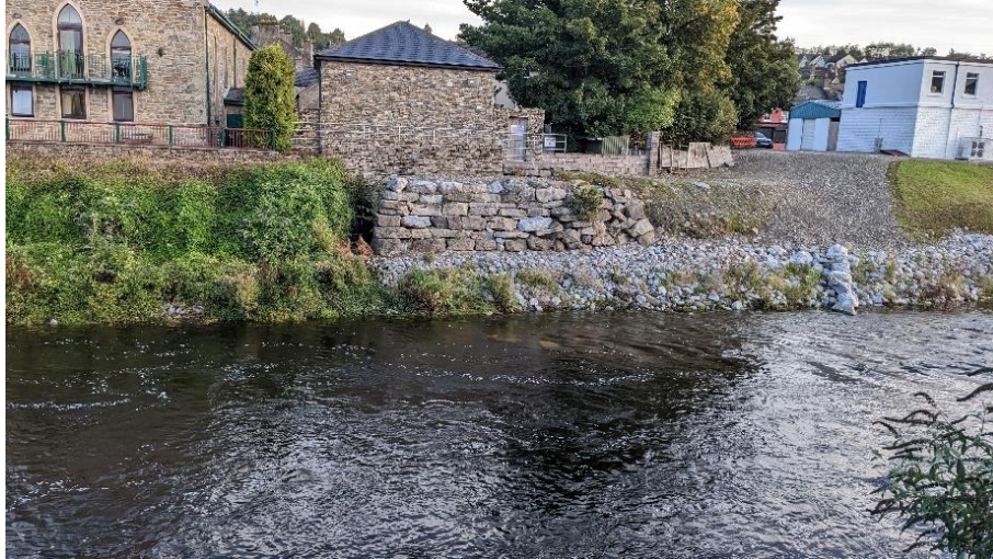
Figure 5.4 Watergate Street PS SWO/EO SW004
