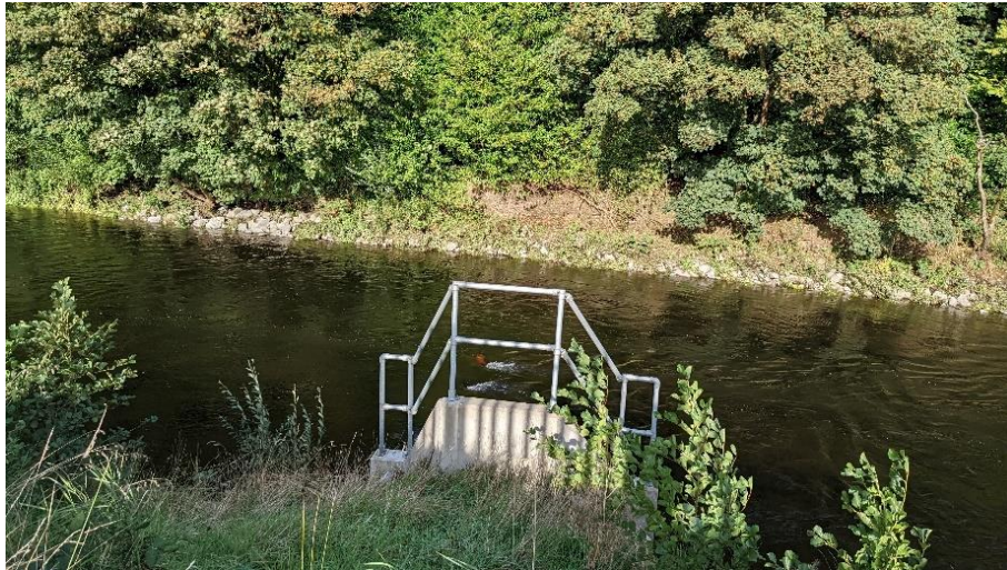
Figure 5.5 WwTP SWO/EO SW002
