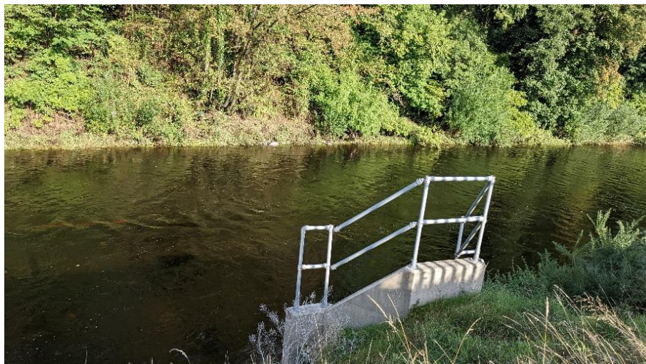
Figure 5.7 WwTP Primary Discharge SW001
