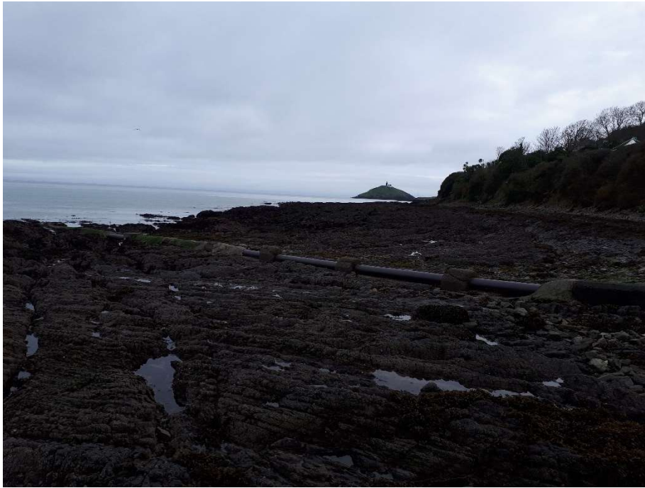
3 - Outfall pipe downstream of existing septic tank
