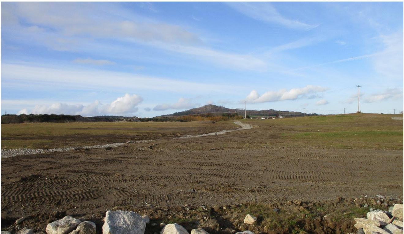
Plate 4 – View Looking North along Recently Completed Land Drain
