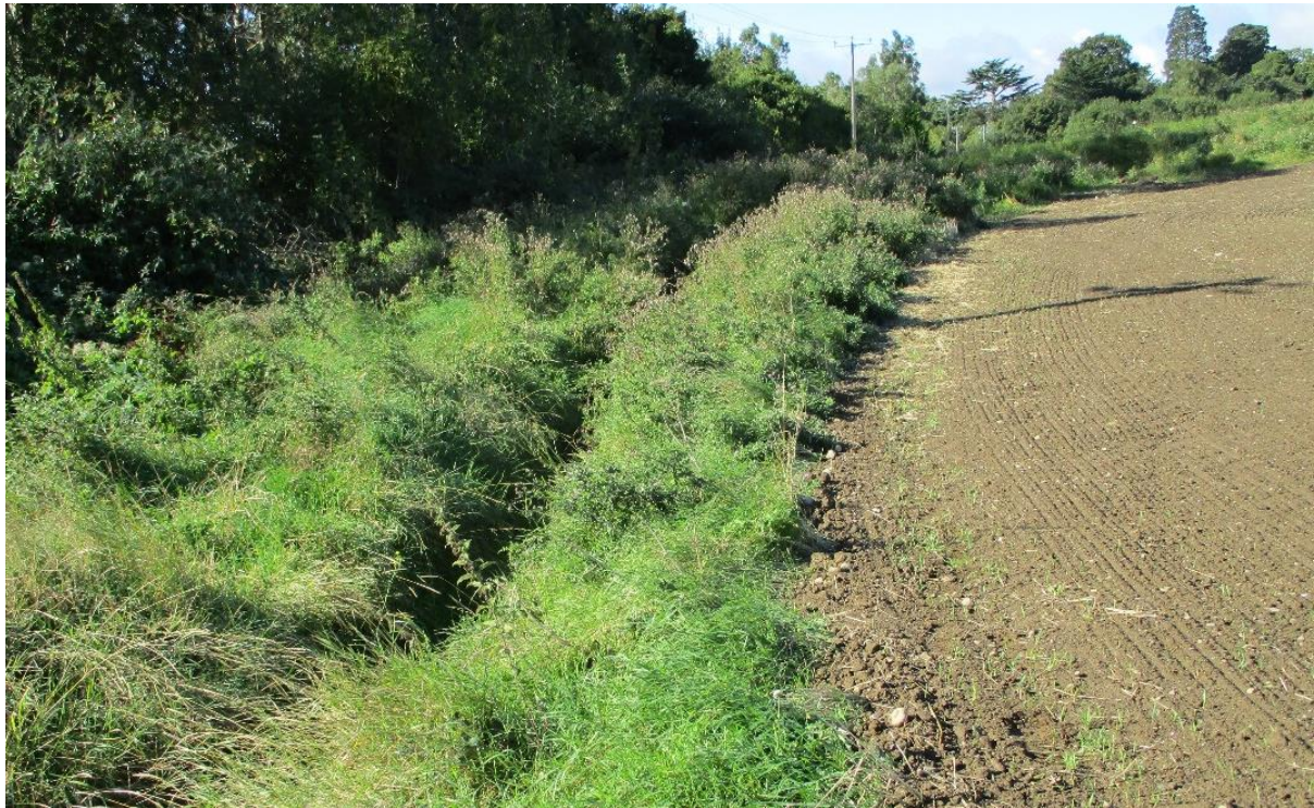
Plate 5 – View Along Existing Channel Leading from Backfilled Area to Manhole
