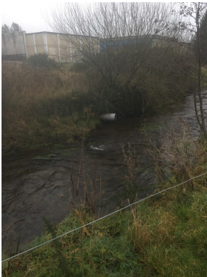
Figure 4.3 Pipe from industrial unit
