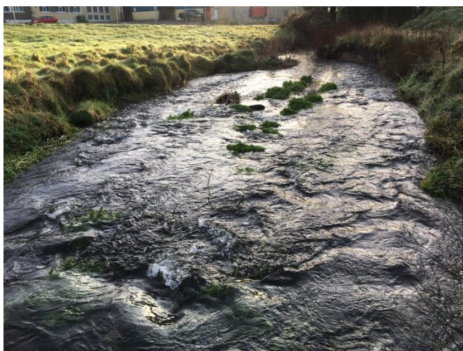
Figure 4.2: Downstream of primary discharge Grenagh WWTP
