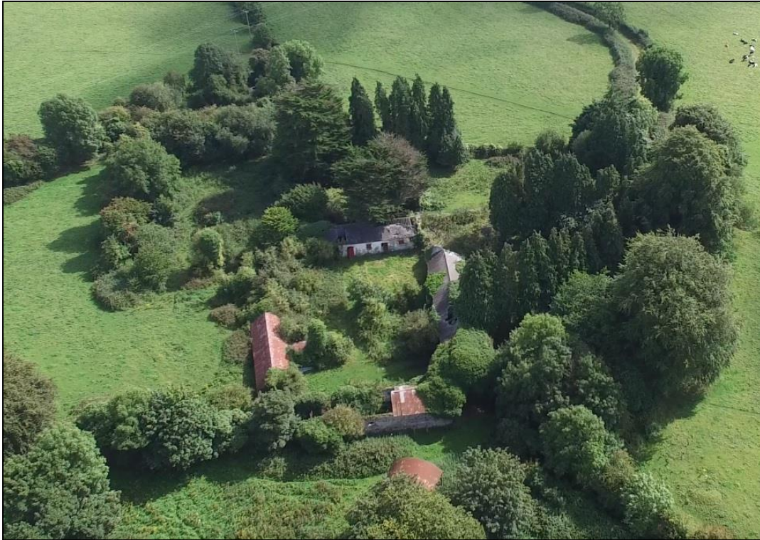
FIGURE 4.22 NEVINSTOWN HOUSE AND OUTBUILDINGS
