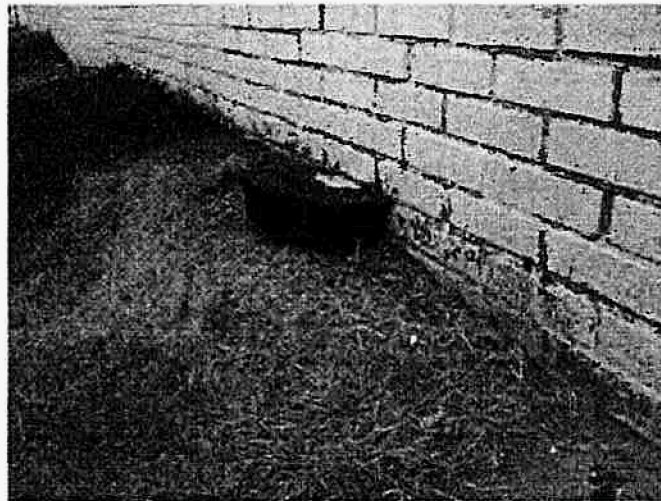
Figure 2. Rat bait station properly placed against the exterior wall of a building.
