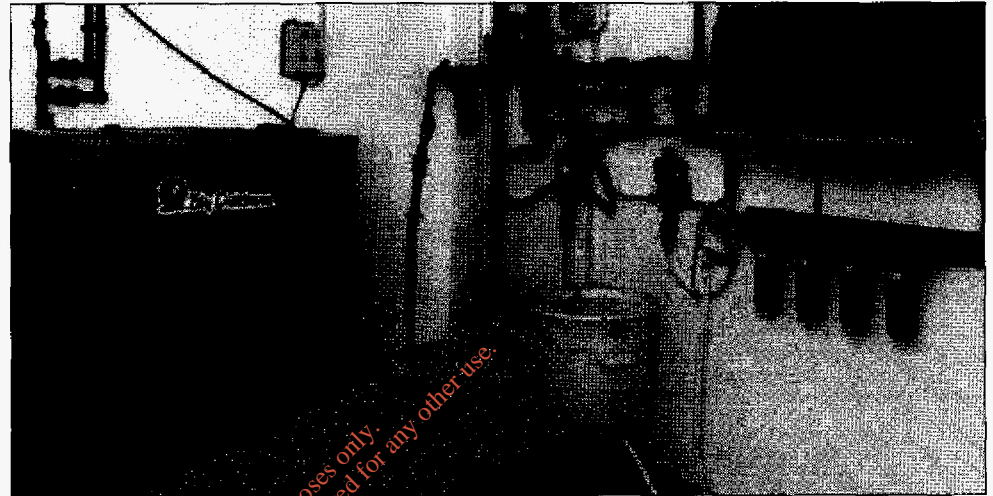
Service room with small and large mixing tank for medicines
