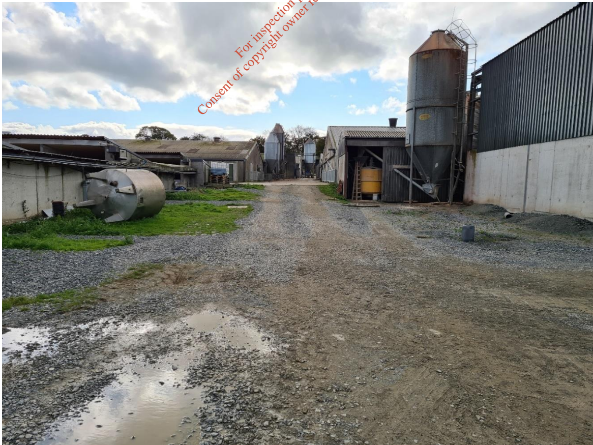
Plate 9: Buildings 3-11 on left-hand-side and mill and buildings 13-15 on right-hand-side
