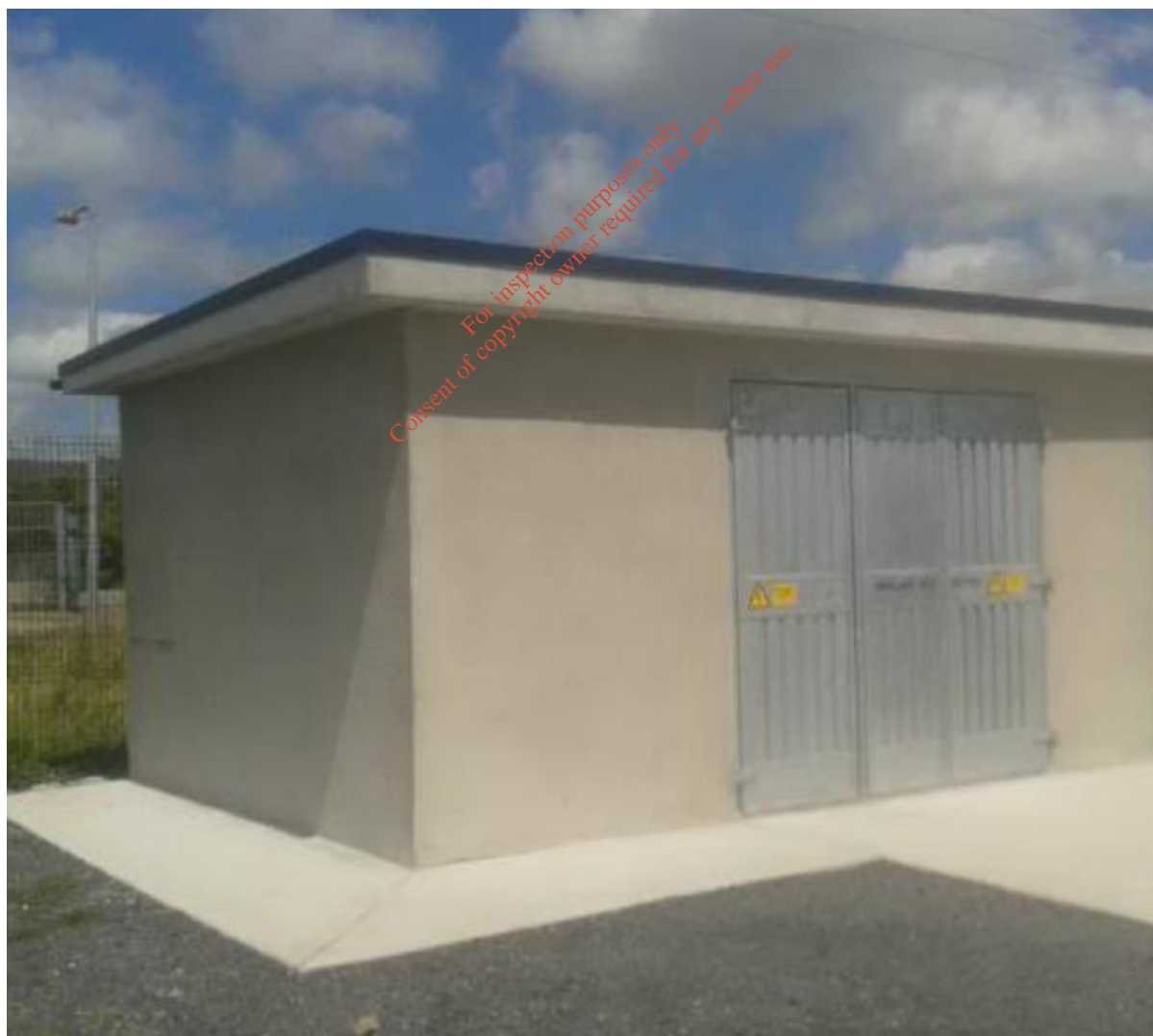
Plate No 1: Example of single mv electrical substation
