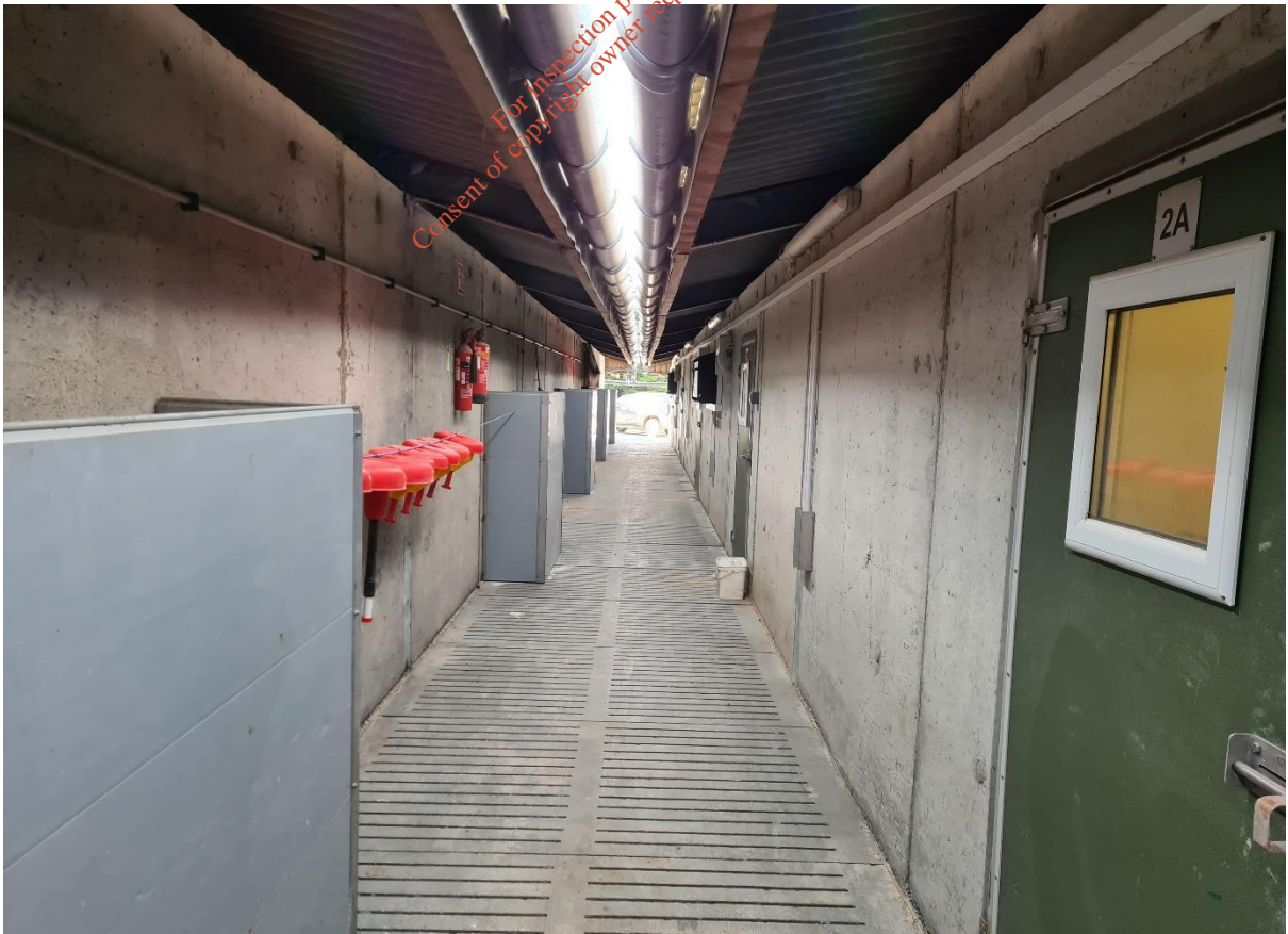
Plate 5: Covered slatted pig-walk passage.
