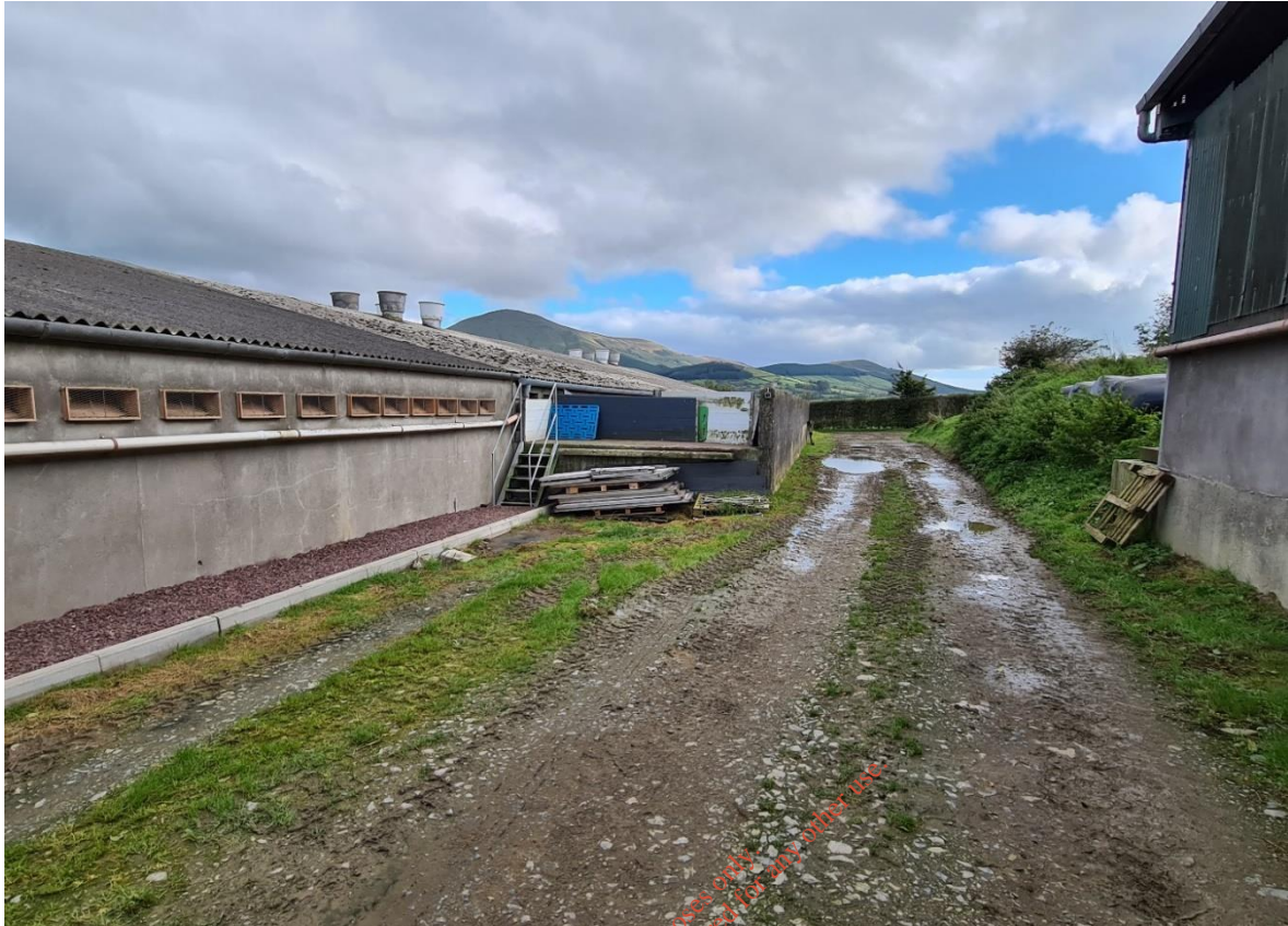
Plate 8: Building No 11 on Left-hand-side and looking SE onto loading bay
