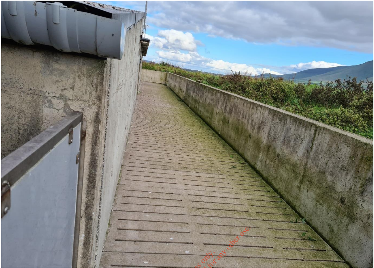
Plate 6: Un-covered slatted pig-walk passage
