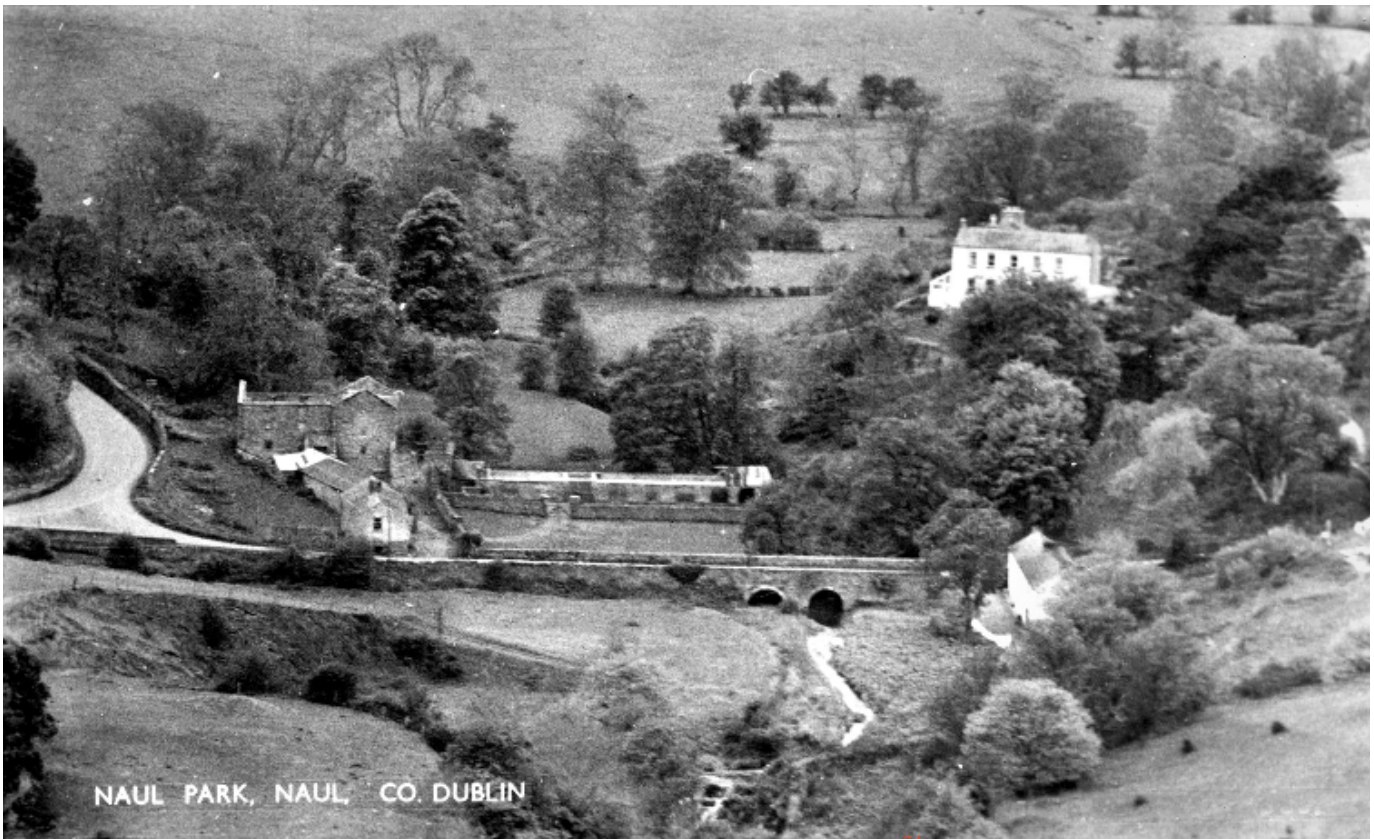
Naul Bridge c.1930 showing location where parapet was removed for access to the treatment plant site.
