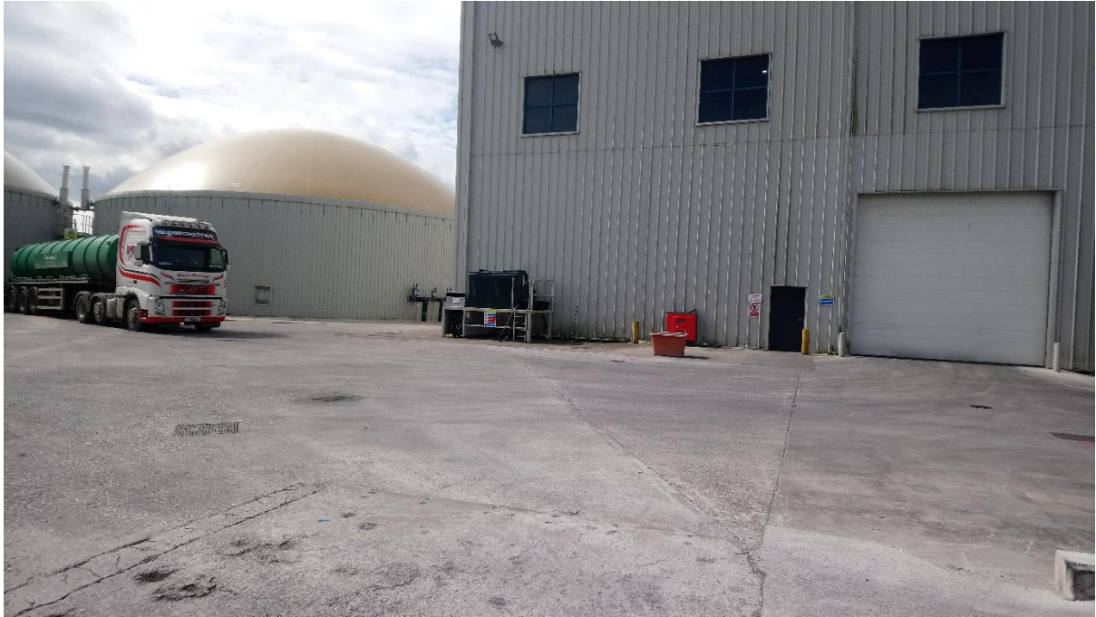
Photograph 1: Diesel Storage Tank Building 1
