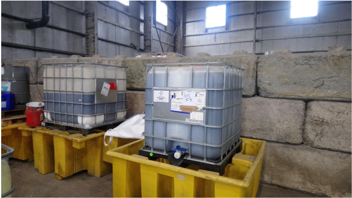
Photograph 3 : Engine and Hydraulic Oil
