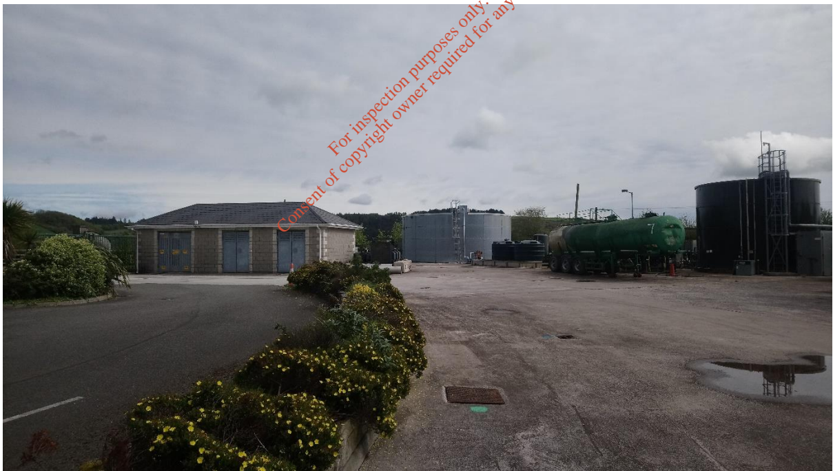
Photograph 8; Electrical Substation and Firewater Storage Tank
