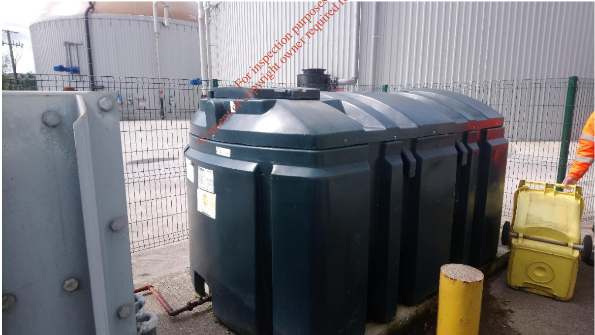
Photograph 2: Diesel Storage Tank Building 2
