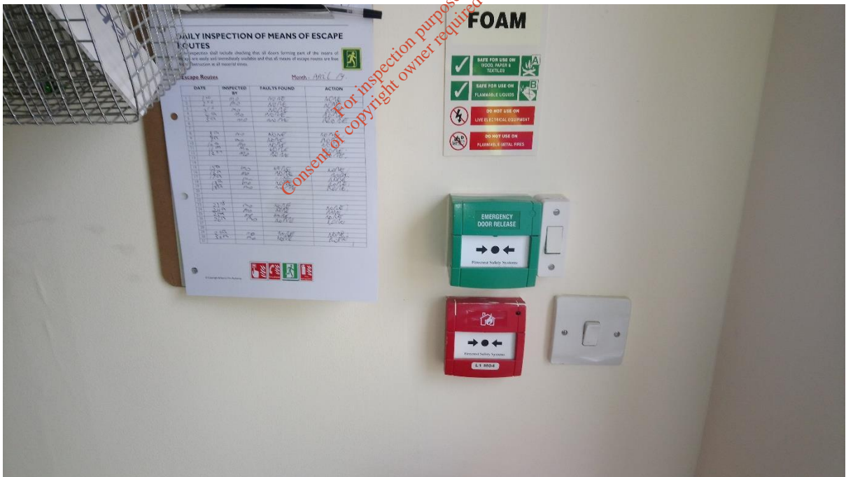
Photograph 6: Emergency Break Glass, Door Release and Exit Inspection Sheet-Office
