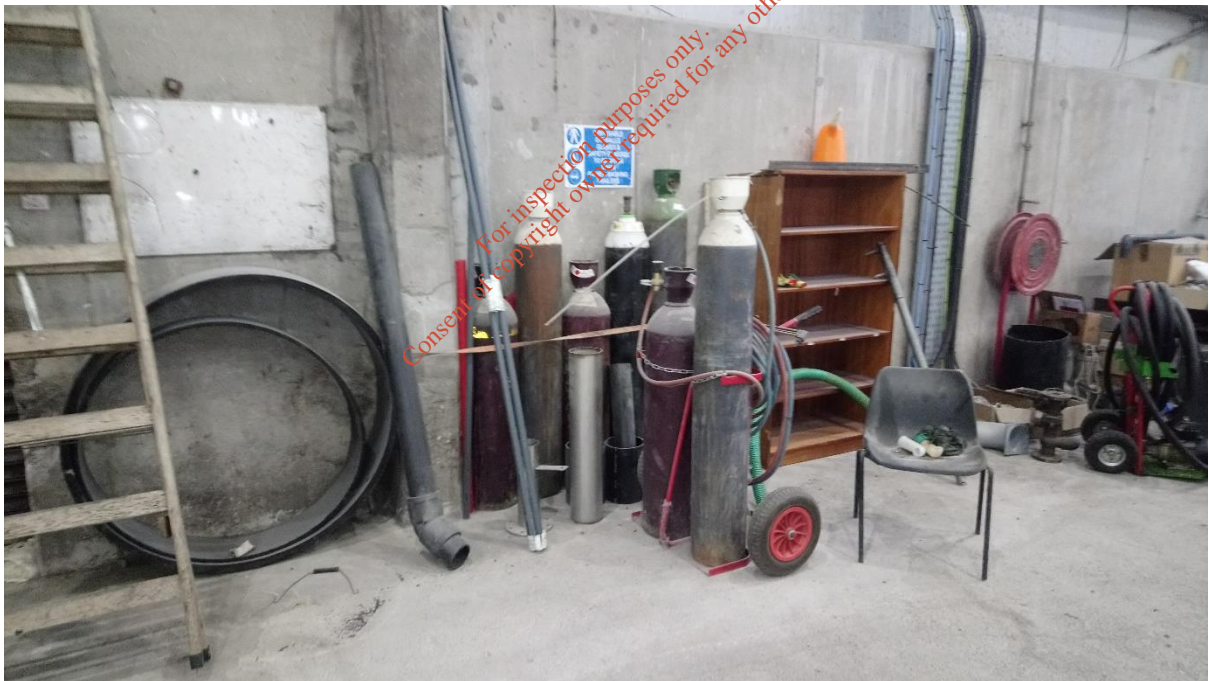
Photograph 4 : Gas Cylinder Storage
