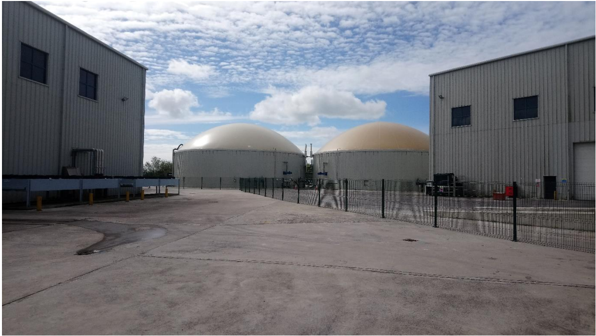
Photograph 9: Building 2 on left, digesters in centre and Building 1 on right
