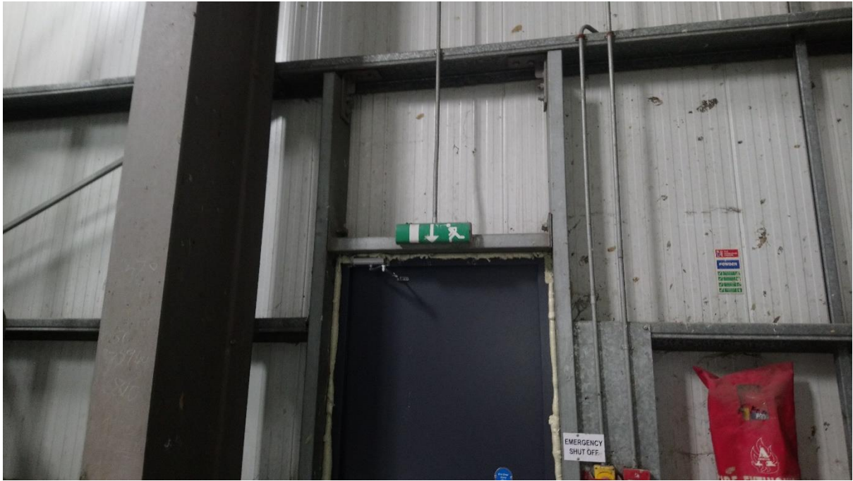
Photograph 31 : Emergency Exit Door Building 2
