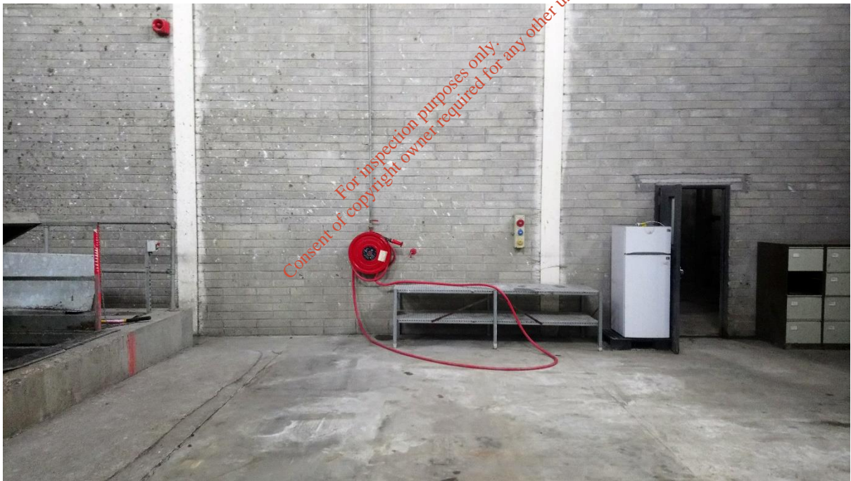
Photograph 32 : Hose Reel Building 2
