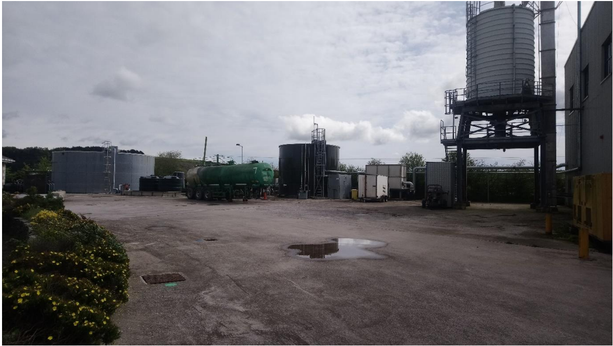
Photograph 7 WWTP and Sludge Silo
