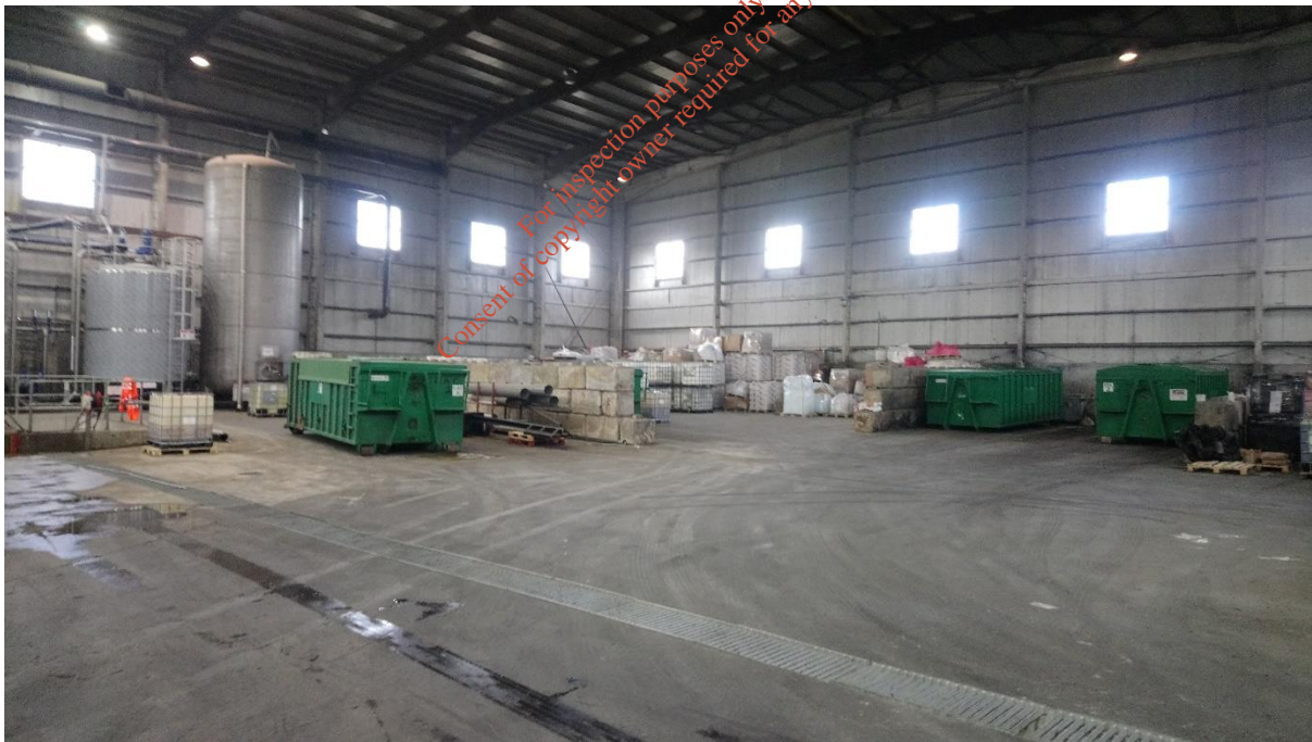
Photograph 6: IBC Storage Building 1
