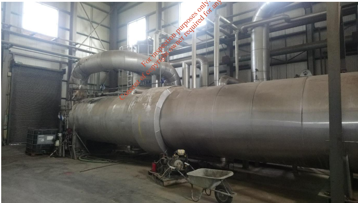
Photograph 30 :Rotary Drier Building 2
