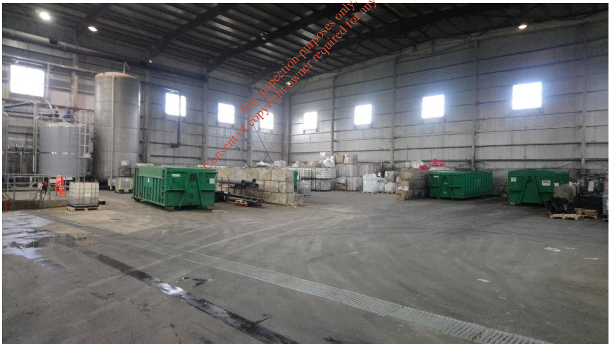
Photograph 22 : Waste Storage Bays Building 1
