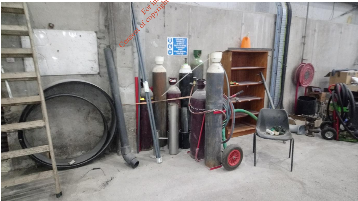
Photograph 26 : Gas Bottle Storage Building 1
