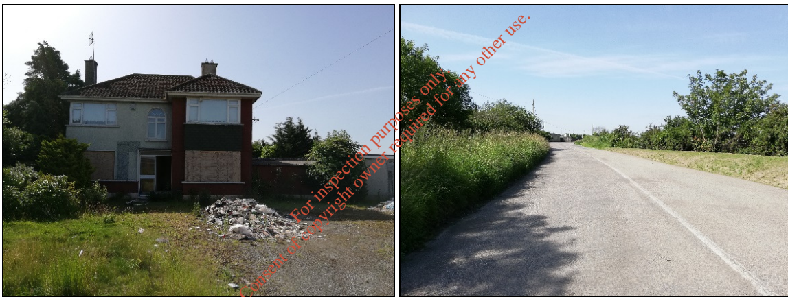
Figure 6.7 Buildings and artificial surfaces (BL3) occurring within the Proposed Development site
