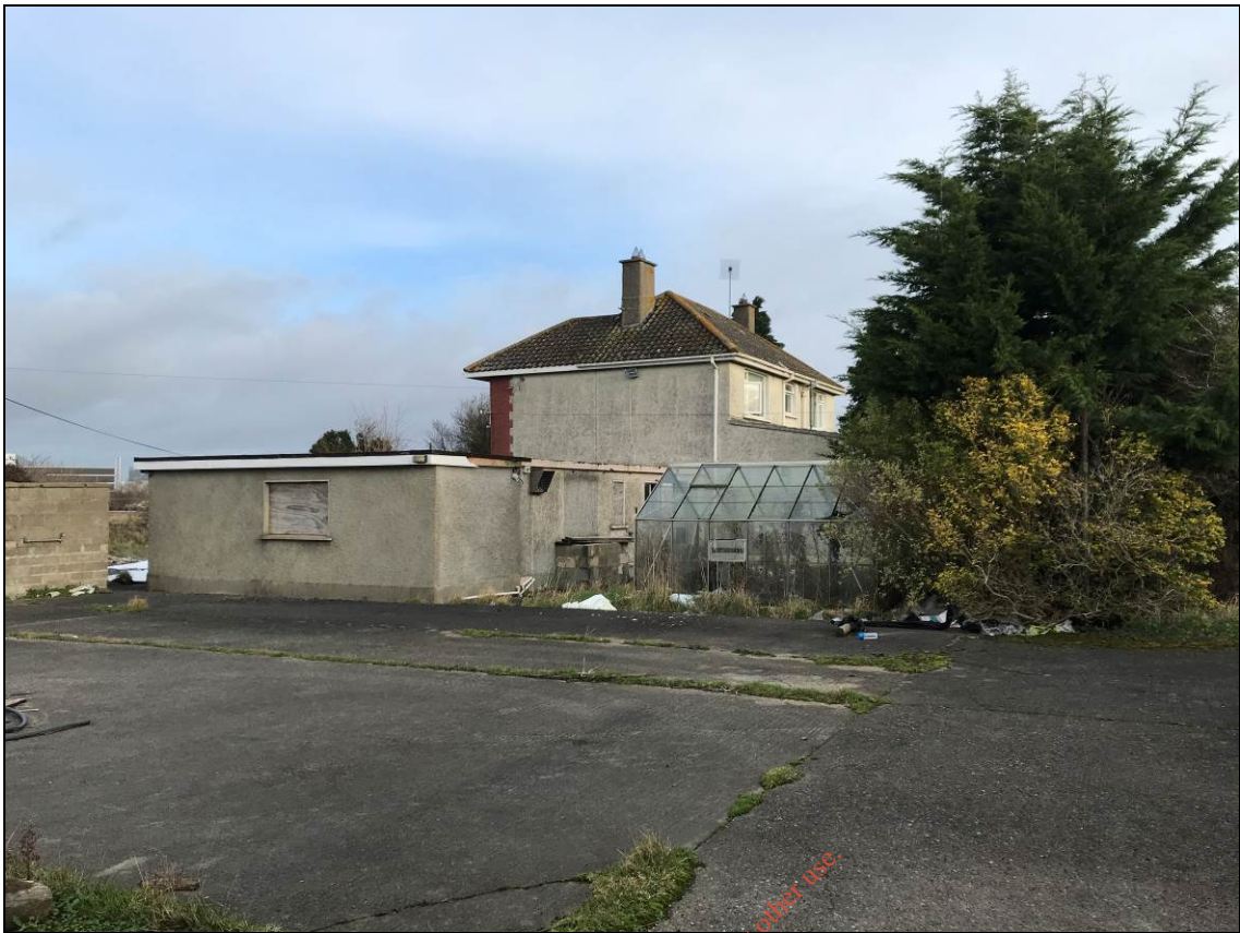
Figure 13.11 Farm house, facing northeast
