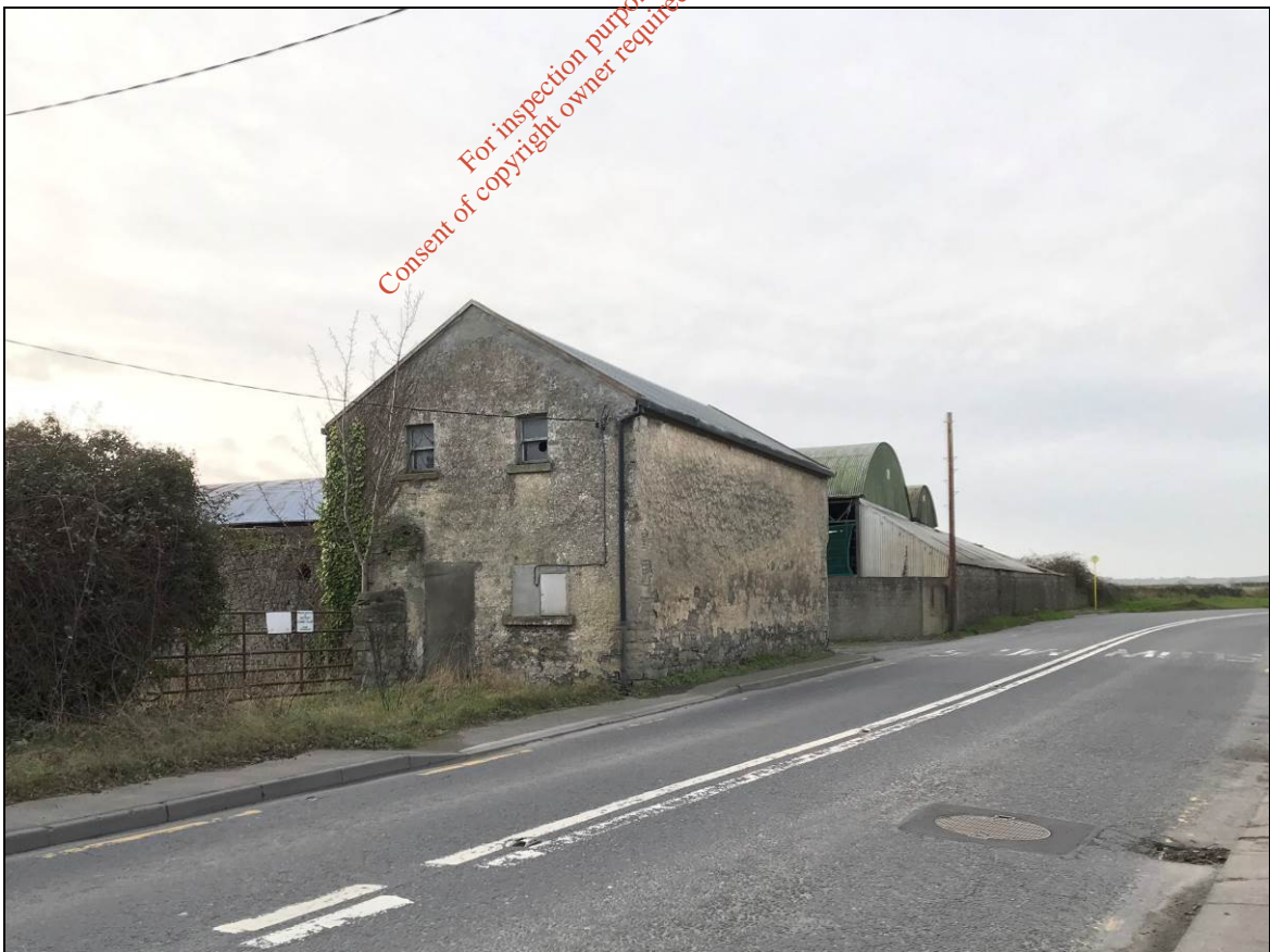
Figure 13.16 Outbuilding (NIAH Ref. 11208006), facing southeast
