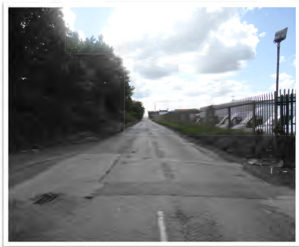
Plate 13-4 Kilshane Road near western quarry entrance
