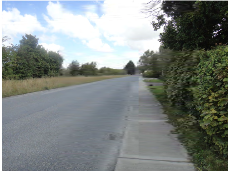
Plate 13-3 North Road near quarry entrance
